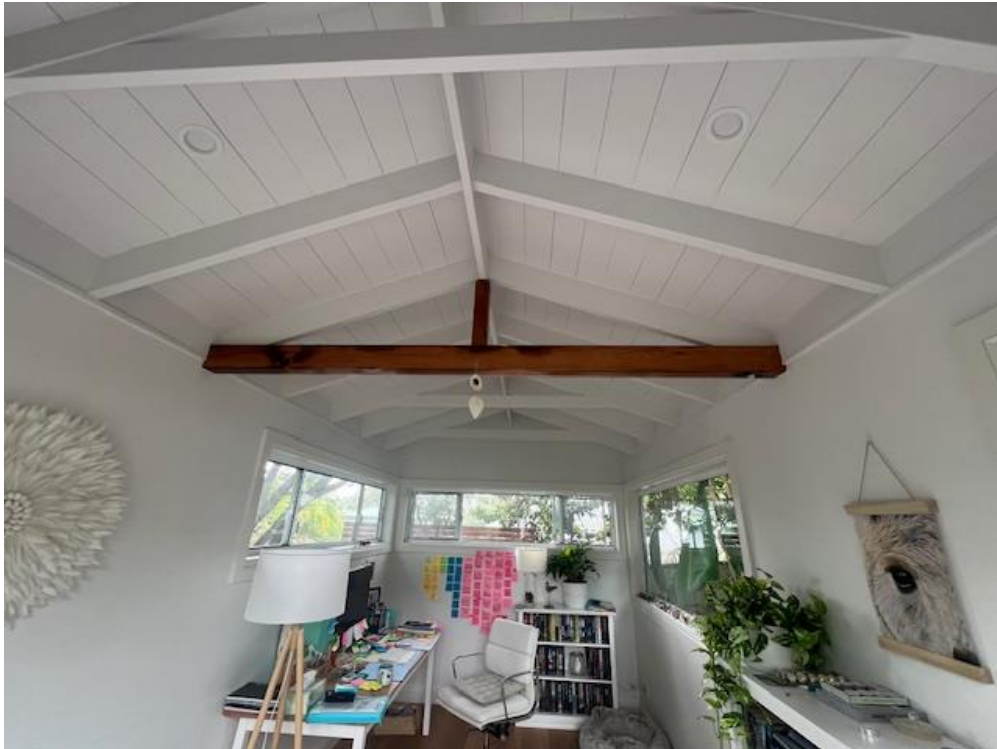
Photo 1: Existing conditions of studio roof framing
