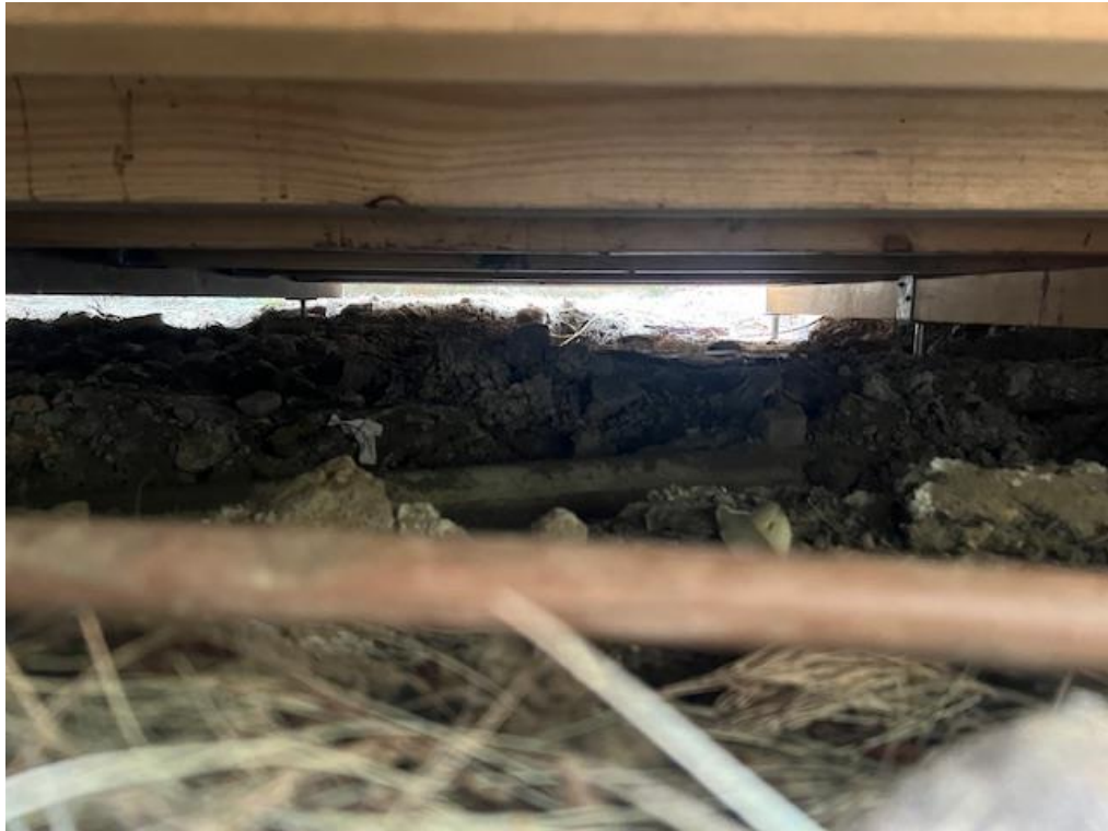
Photo 3: Existing conditions of studio floor joists
