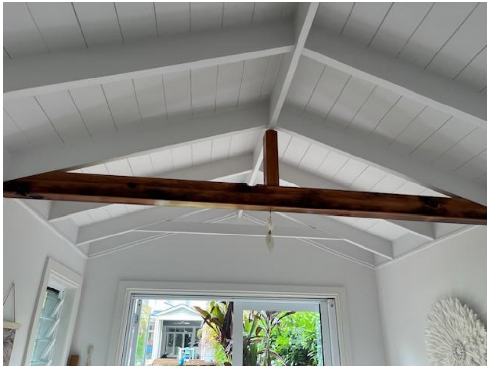
Photo 2: Existing conditions of studio roof framing & opening
