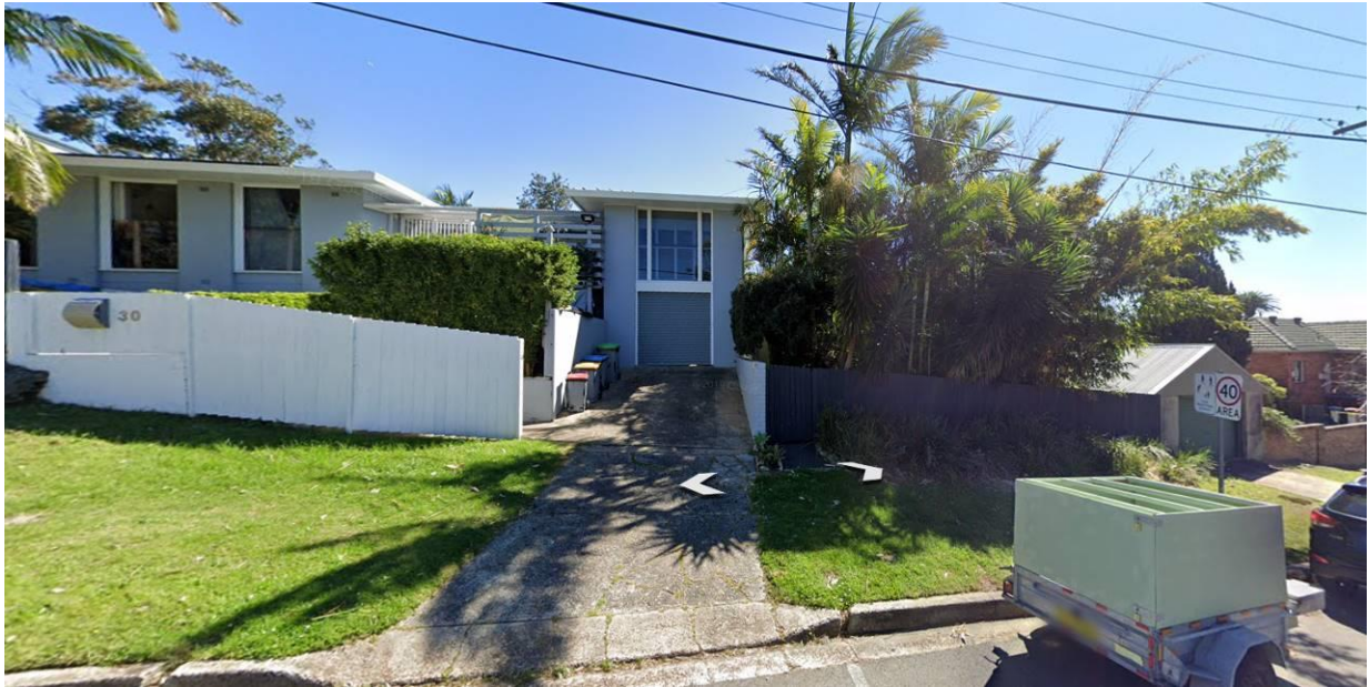
Figure 8: Adjoining dwelling house to the south as viewed from Dowling Street
