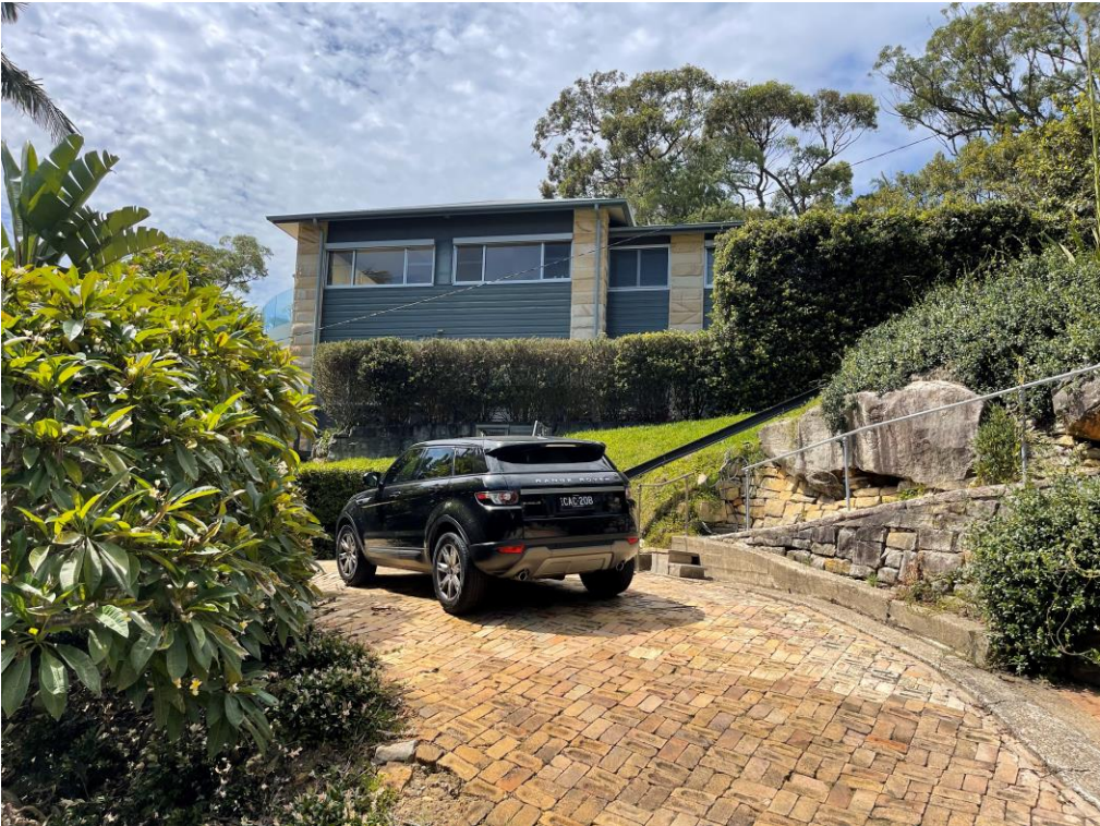
Fig 6: View of the existing parking area and location of new carport with studio above, looking east
