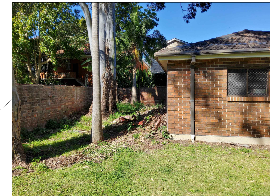
EXISTING BRICK MASONRY ALONG EASTERN BOUNDARY TO BE RETAINED AND REPAIRED FOR REUSE
