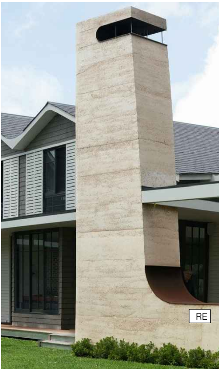
rammed earth chimney
