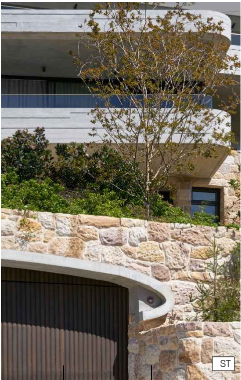
sandstone retaining walls + garage door
