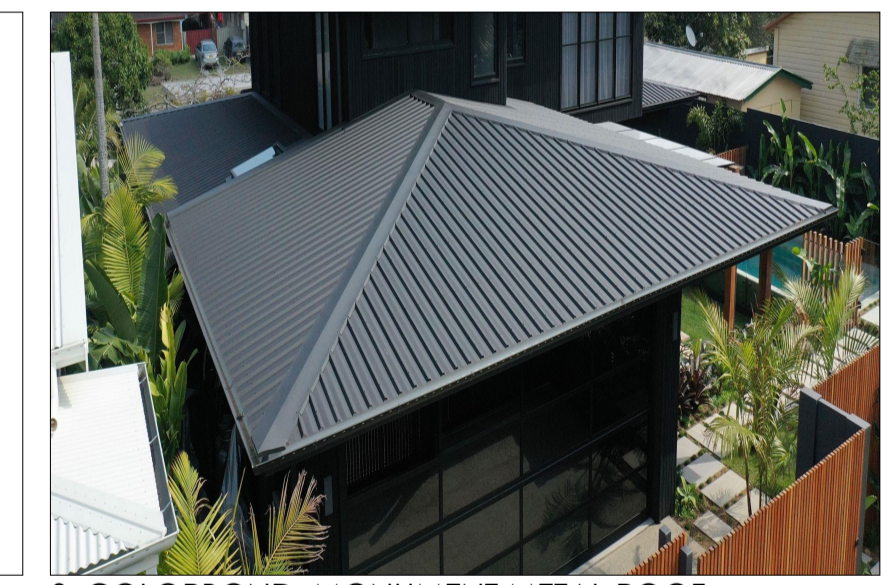
3. COLORBOND MONUMENT METAL ROOF
