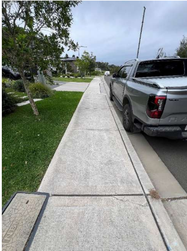
Figure 31 – Crack is evident to the footpath outside of 59 Lorikeet Grove Warriewood
