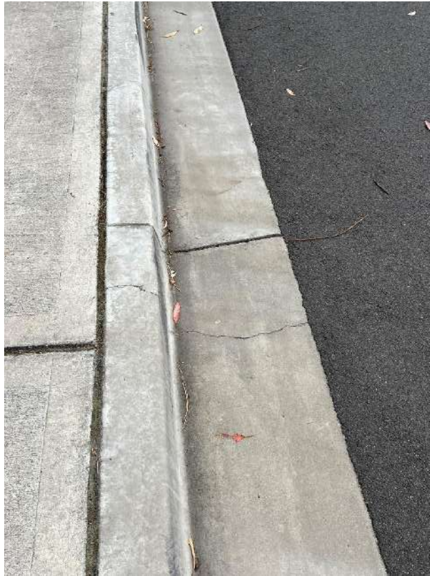
Figure 15 – Crack is evident to the kerb at the opposite side of 57 Lorikeet Grove, Warriewood.
