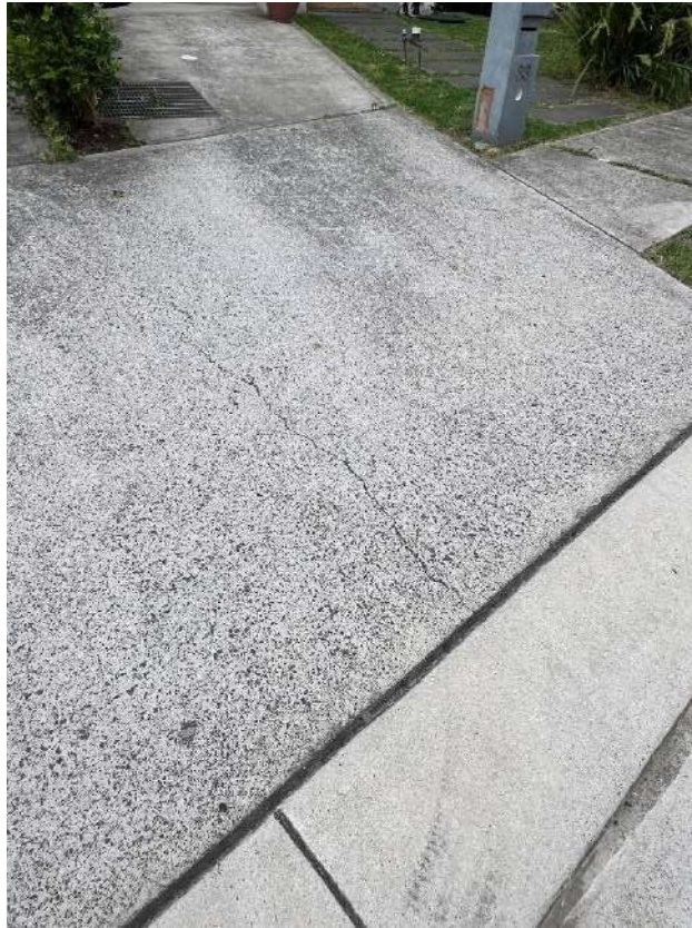
Figure 59 – Crack is evident to the driveway outside of 33 Lorikeet Grove, Warriewood
