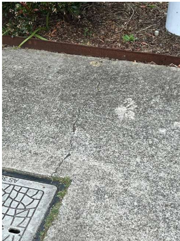
Figure 58 – Crack is evident to the footpath outside of 31 Lorikeet Grove, Warriewood
