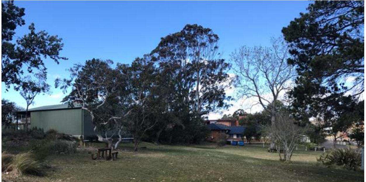
Figure 3 Looking east at the existing buildings on the eastern portion of the site
