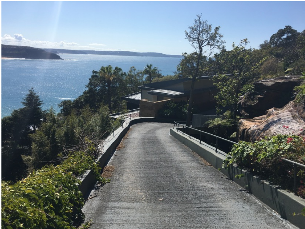
Figure 8: The shared driveway leading to No. 15 Florida Road. The subject cottage is situated below the driveway.
