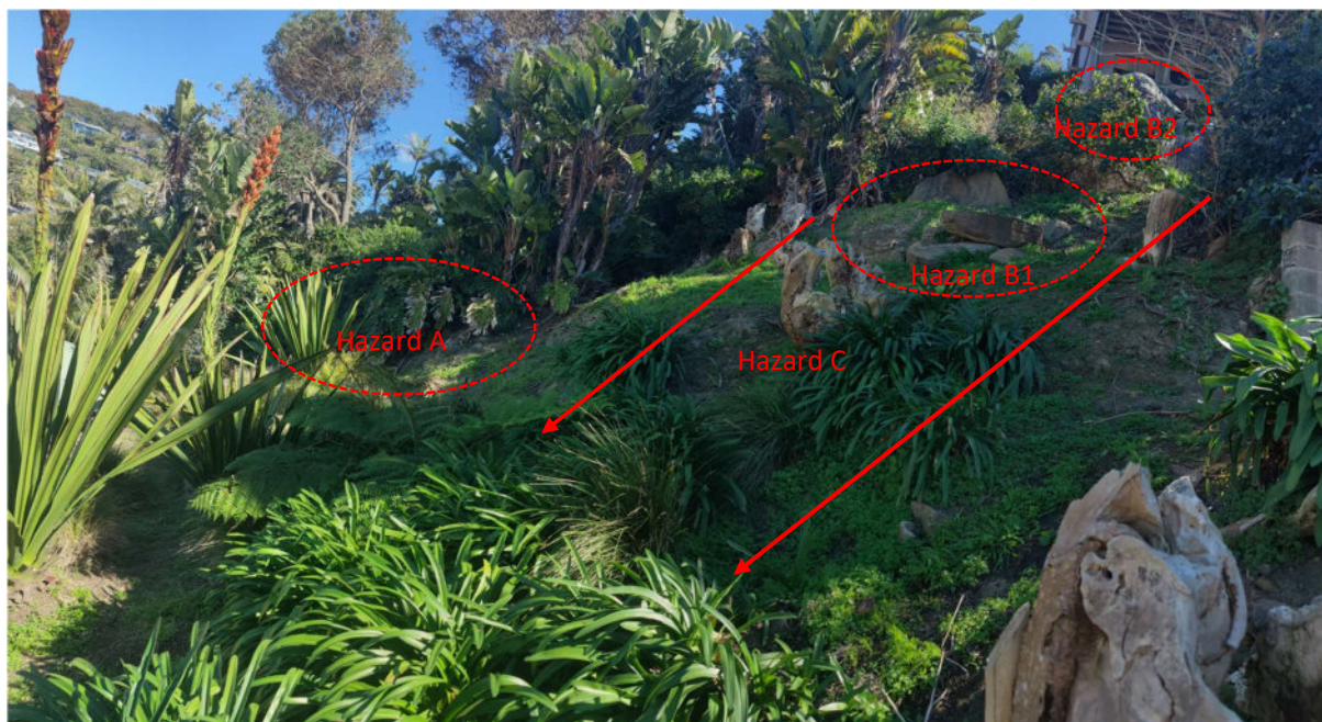
Plate 2 - Hazard A, B1, B2 and C (2 Photographs) – Taken from downslope
