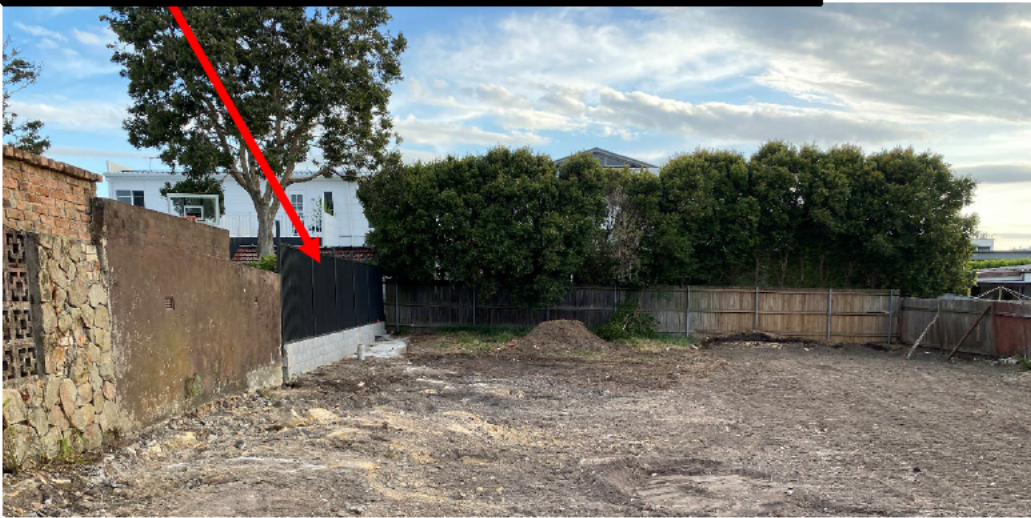
Figure 3: Completed portion of the dividing fence, viewed from No. 1 Summit Ave.
