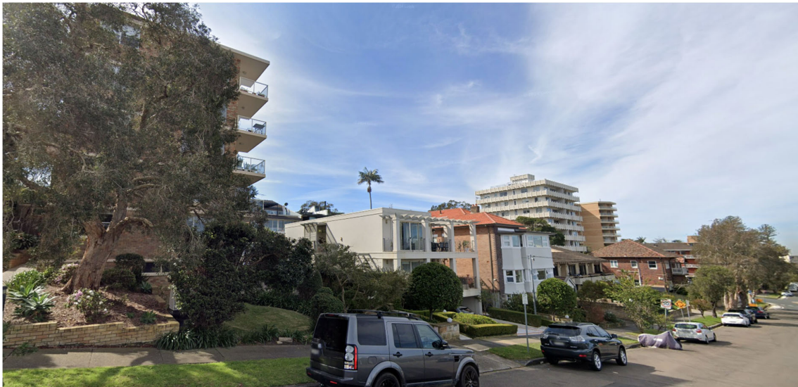
The existing streetscape on northern side of Fairlight St (Google Maps)
