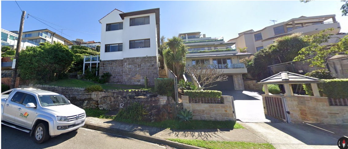
Existing site at 10-12 Clifford Avenue (Google Maps)
