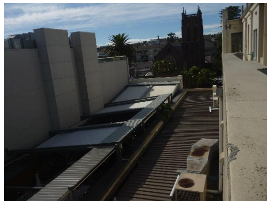
Figure 13: Rooftop view of 25 and 23 The Corso looking towards The Corso frontage
