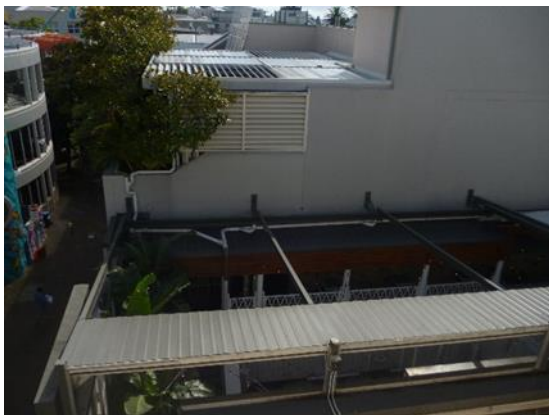
Figure 12: Rooftop view of 25 The Corso showing Market Place section
