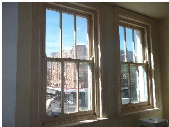
Figure 21: Original Timber framed windows at 19-21 The Corso.
