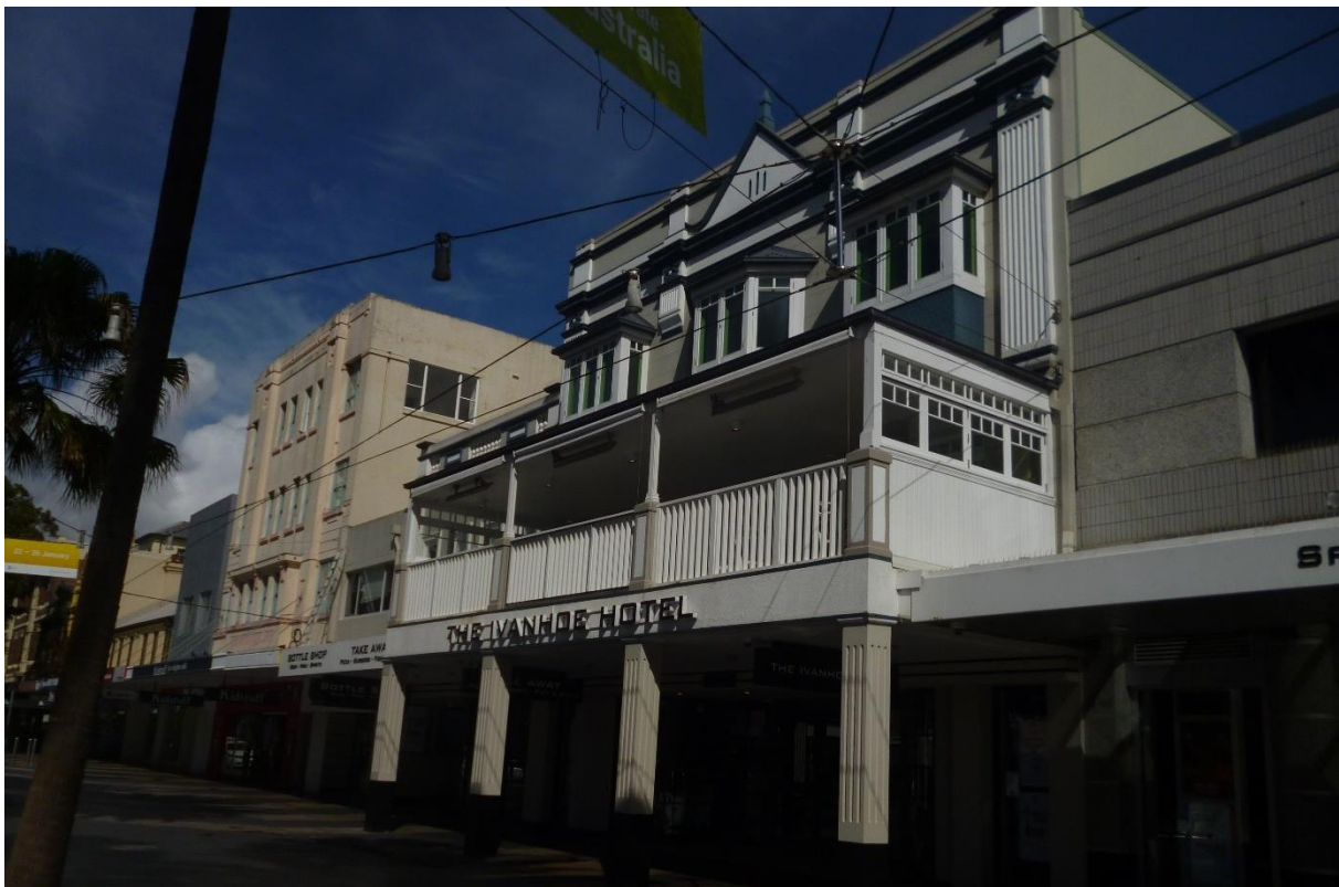
Figure 23: Front elevation of The Ivanhoe Hotel (27-29 The Corso).
