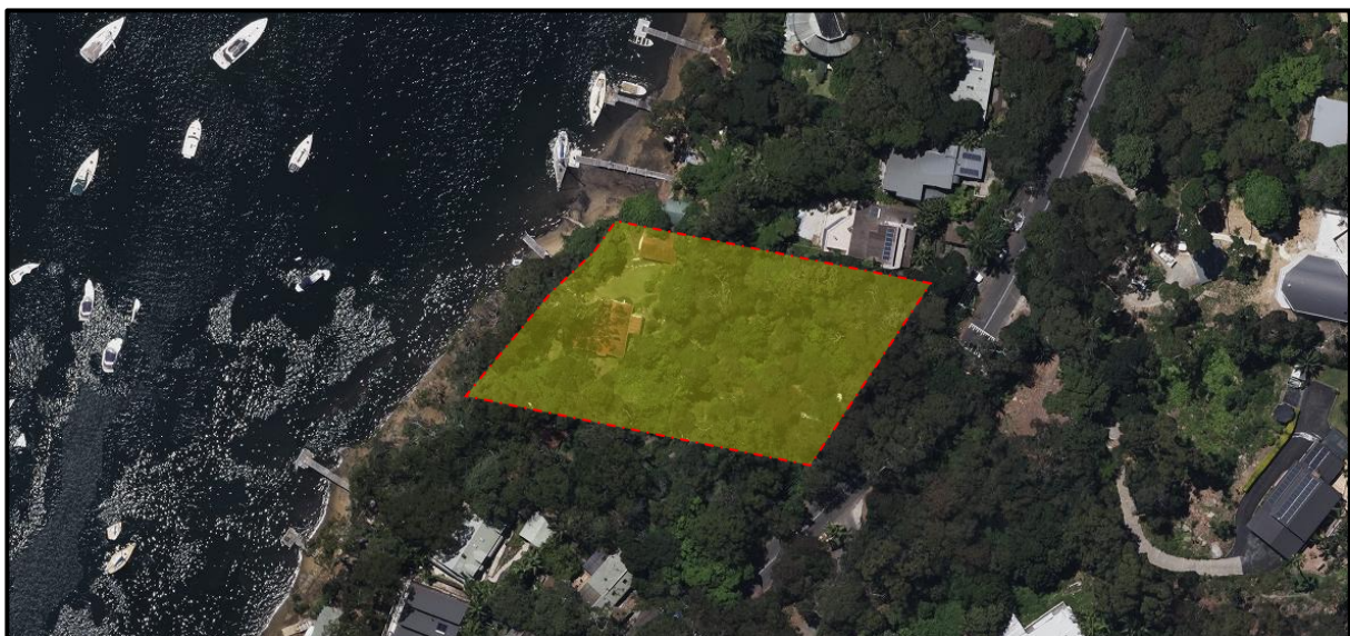
Figure 1. Site location – 158A McCarrs Creek Road, Church Point (© SIX Maps NSW Gov)
