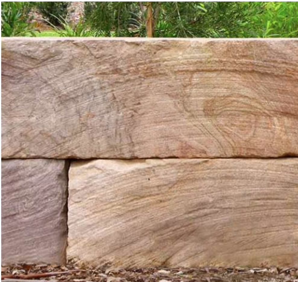
SANDSTONE WALLS TO VERGE
