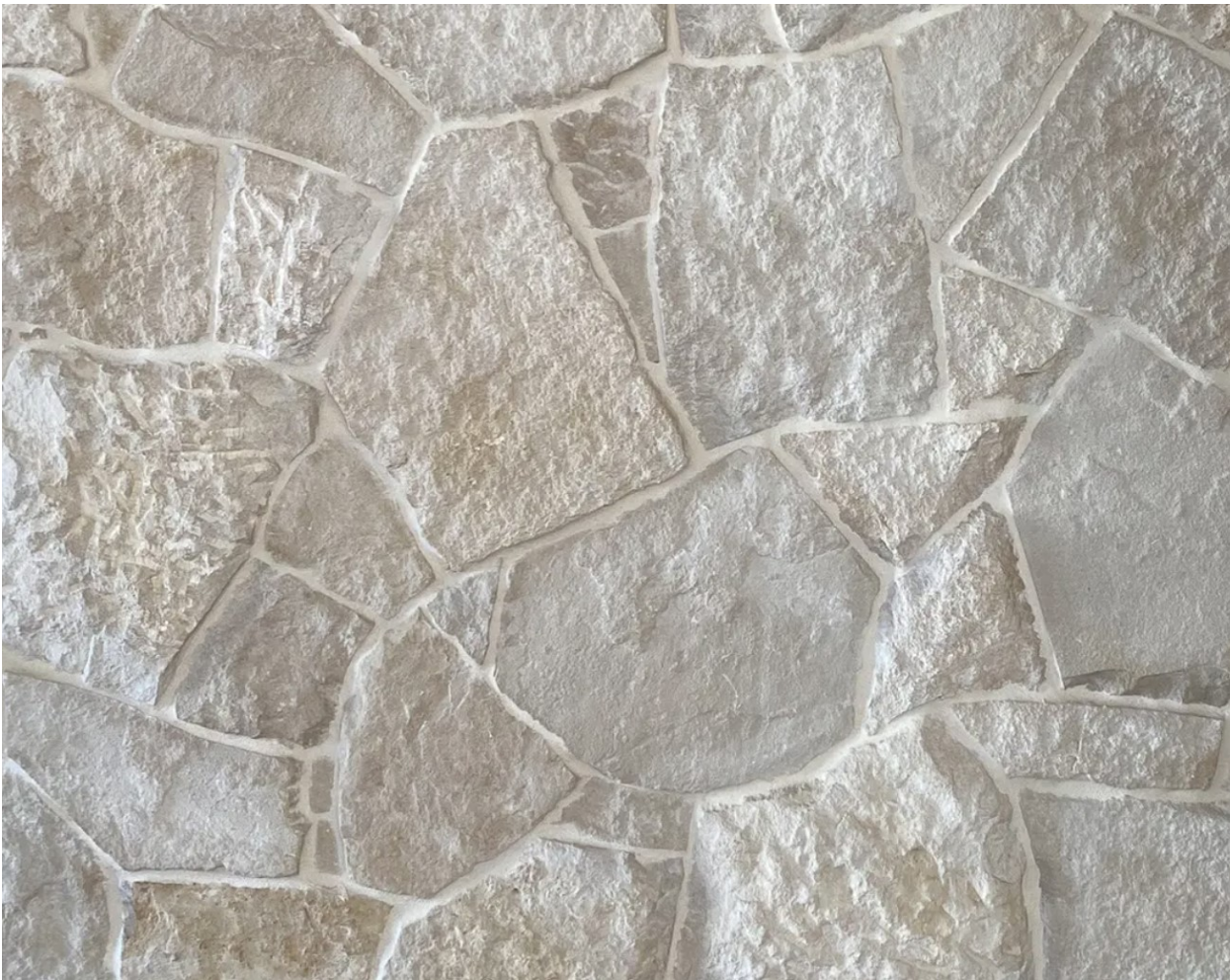
STONE CLADDING TO GARAGE FACADE
