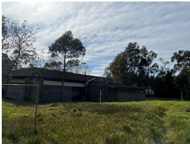
Figure 7: Existing building from Lockwood Avenue side
