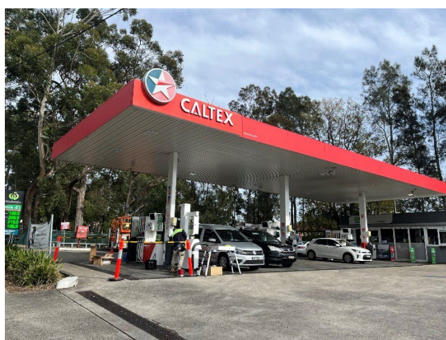
Figure 14: Petrol station to adjoining the site to the east
