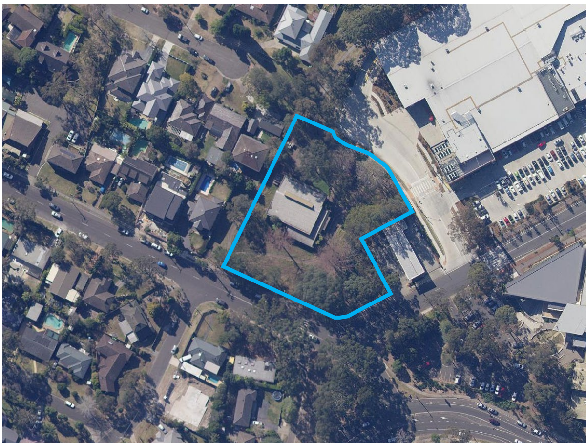
Figure 1: The site and surrounding area
