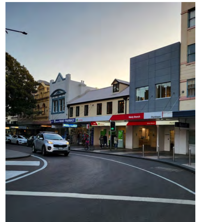
EXISTING SHOPFRONT PHOTOS
