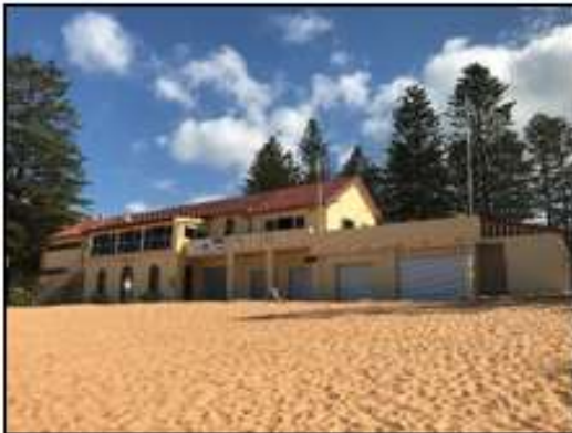
Figure 58. View of the subject building looking from the Northeast edge. (Source: Heritage 21, 23.05.18)
