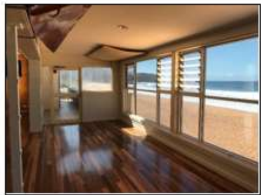
Figure 90. View to the extended covered veranda bay. (Source: Heritage 21, 23.05.18)
