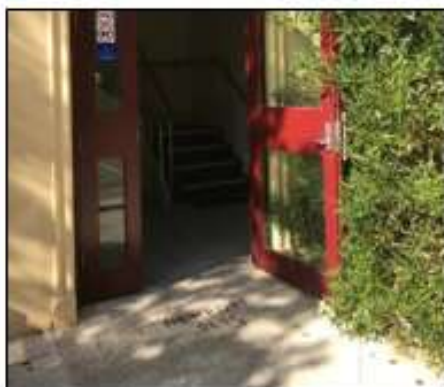
Figure 54. Detail of main entrance, featuring entry threshold with metal letters. (Source: Heritage 21, 23.05.18)
