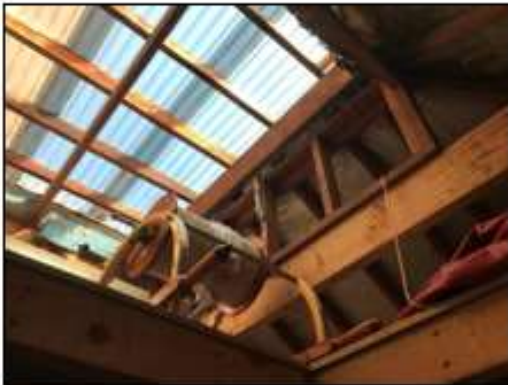
Figure 84. View to roof and timber batons and rafters. (Source: Heritage 21, 23.05.18)
