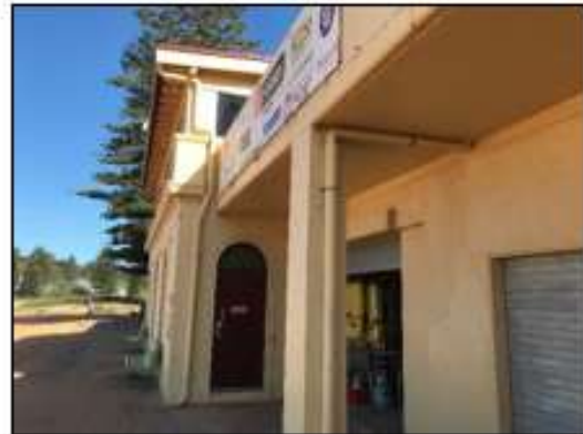
Figure 59. View of the door leading into the first aid room on ground floor and verandah of storage yards. (Source: Heritage 21, 23.05.18)
