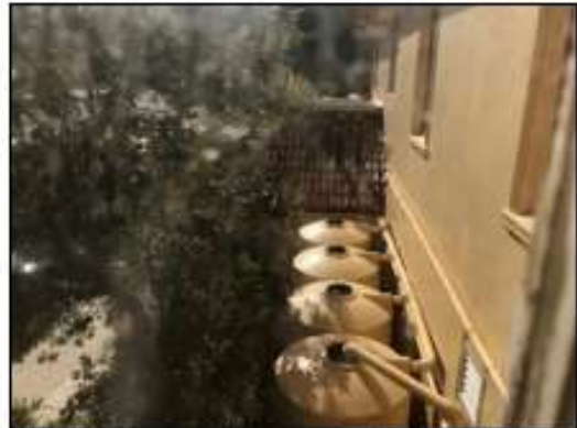
Figure 101. View to the Western elevation from a window in the office above the entry portico. Note water storage tanks and northern wing beyond. (Source: Heritage 21, 23.05.18)
