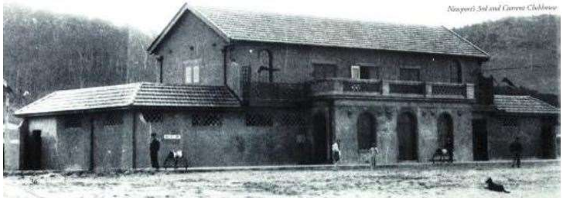
Figure 26: Third and current Newport Clubhouse, built in 1933. 58
