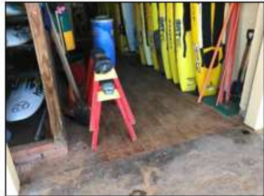
Figure 85. Detail of floor in storage area behind roll-up shutter doors. (Source: Heritage 21, 23.05.18)
