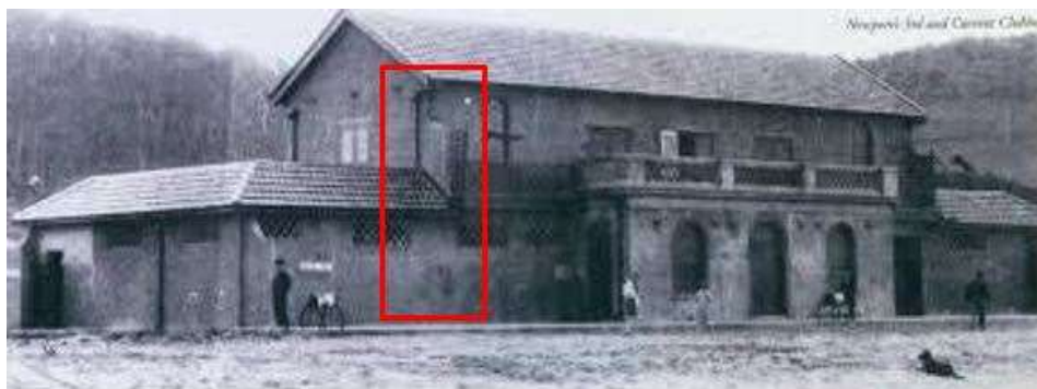
Figure 51 - Photograph indicating original single storey wing alignment with two-storey section walls
