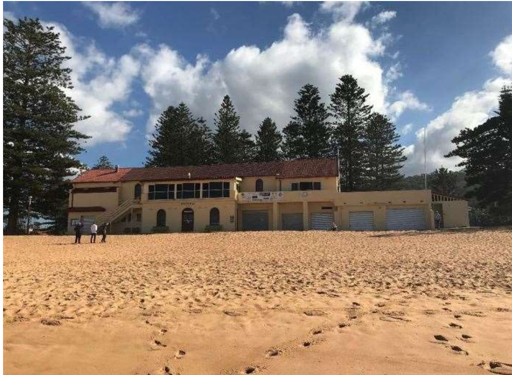
Figure 44: Eastern elevation of the Clubhouse. (Source: Photo taken by Heritage 21, 23.05.18)
