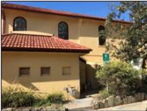
Figure 52. View of the Northern wing. Note the recessed wall between the original and the later addition northern extension. (Source: Heritage 21, 23.05.18)
