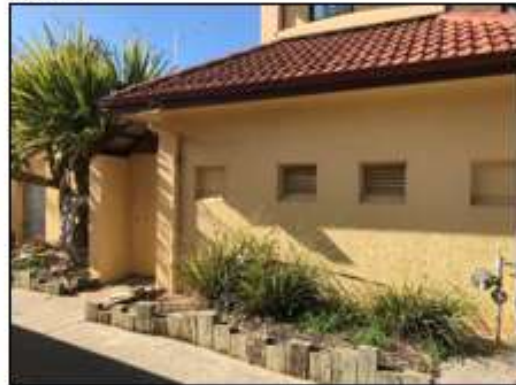
Figure 53. View of the northern wing and side wall that may leads may have led to an earlier entrance to change rooms. (Source: Heritage 21, 23.05.18)
