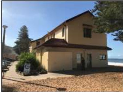
Figure 62. View of the southern wing and extension. (Source: Heritage 21, 23.05.18)
