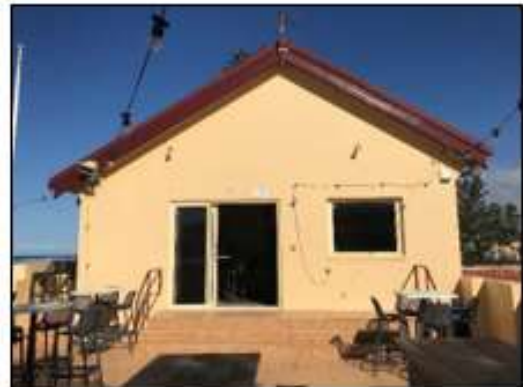
Figure 95. View of the Northern wing from the outdoor seating terrace. (Source: Heritage 21, 23.05.18)
