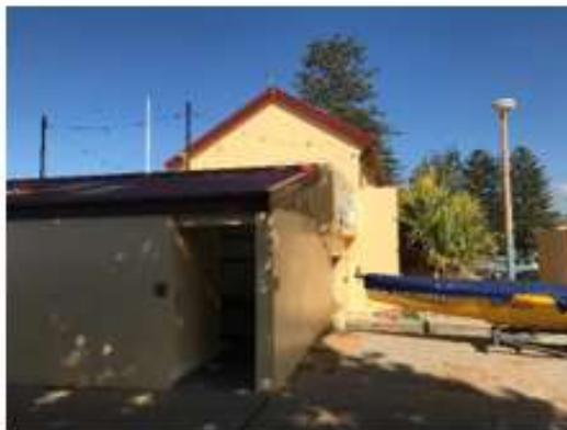
Figure 60. View to the entrance of the public toilets along the northern skillion lean to. (Source: Heritage 21, 23.05.18)
