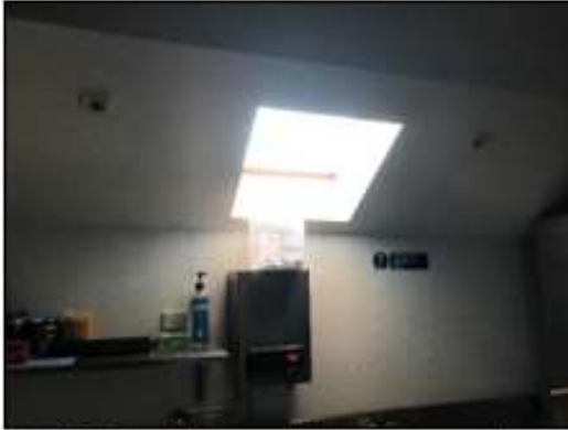
Figure 98. View of the later addition extension covering open to sky areas to facilitate the kitchen. Note modern skylights. (Source: Heritage 21, 23.05.18)
