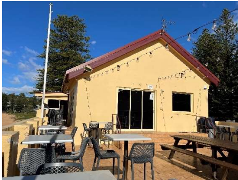
Figure 48: First Floor extension, with terrace area. Note the aluminium access doors and window in the gable wall. (Source: NBRS)
