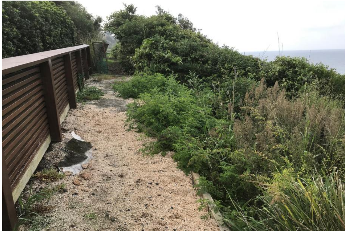
Photo 5: View (looking east) of the gravel pathway at Bilgola Beach Site 1
