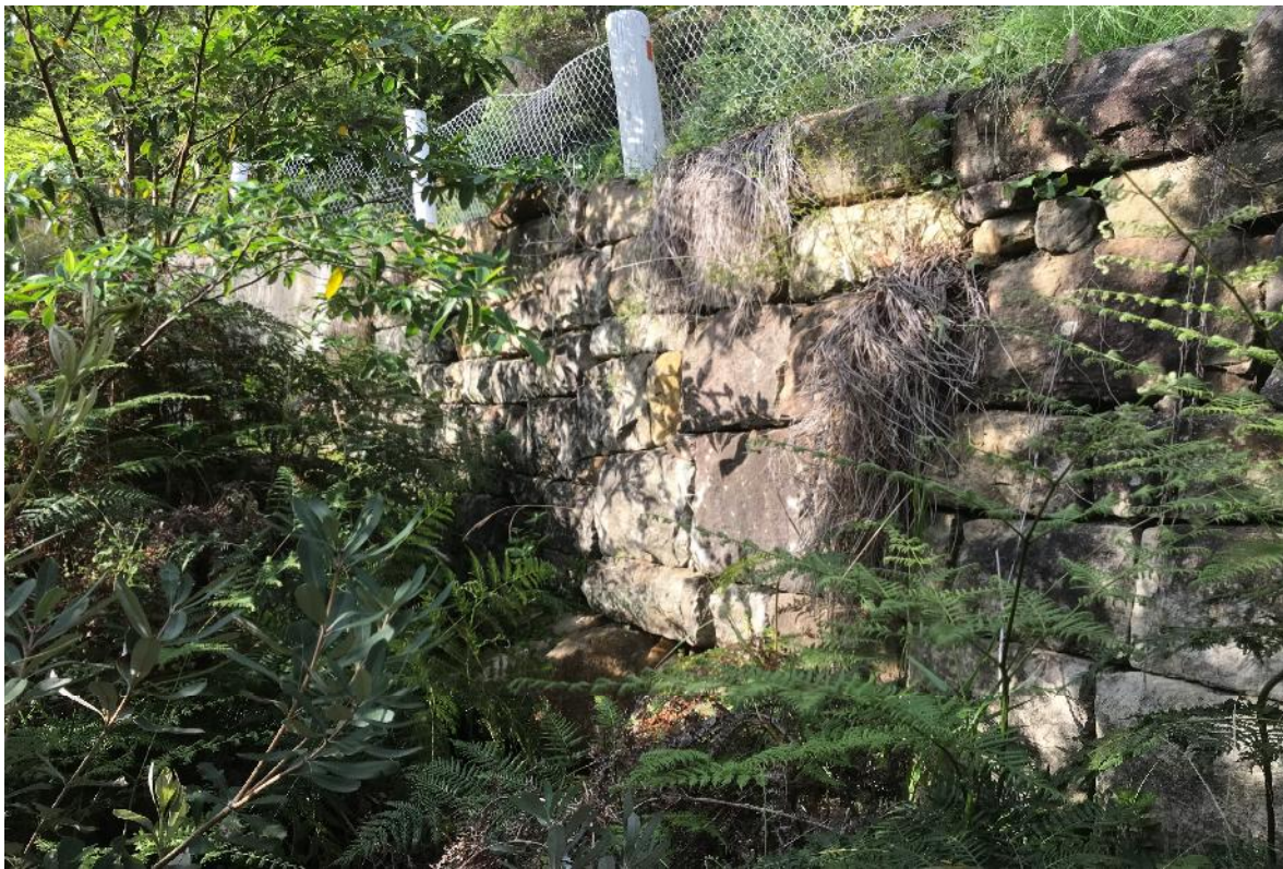
Photo 4: View of a dry-block sandstone retaining wall at Whale Beach Site 1
