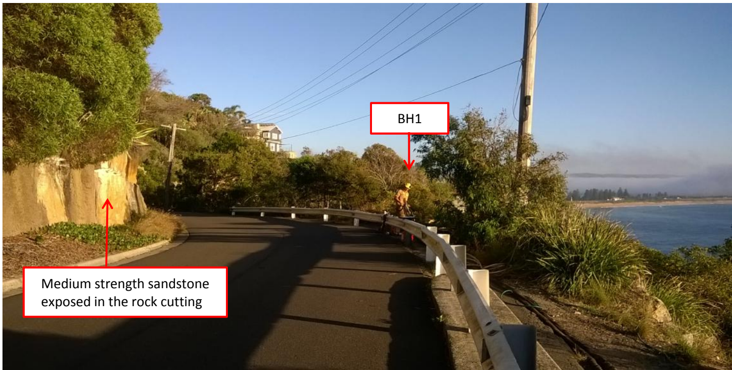
Photo 2: View (looking north) of sandstone cutting on the uphill side of the road
