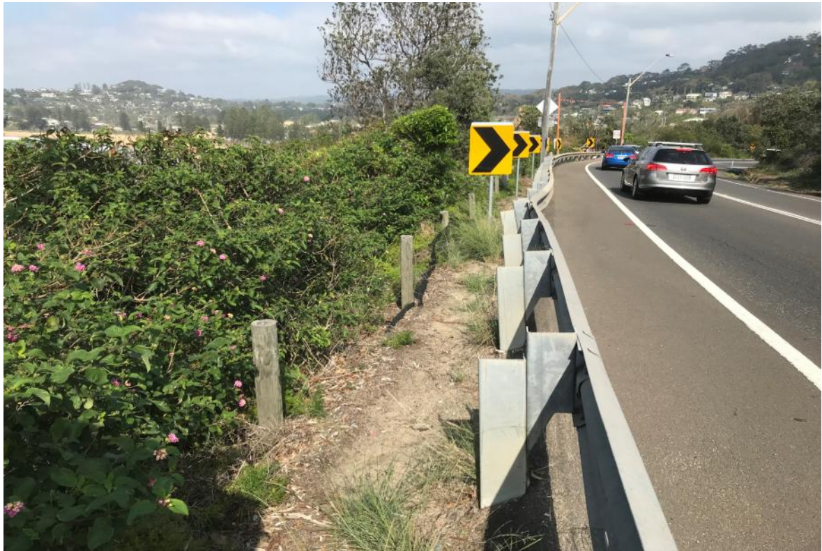
Photo 10: View (looking south) of the Barrenjoey Road embankment at Newport Beach Site 1
