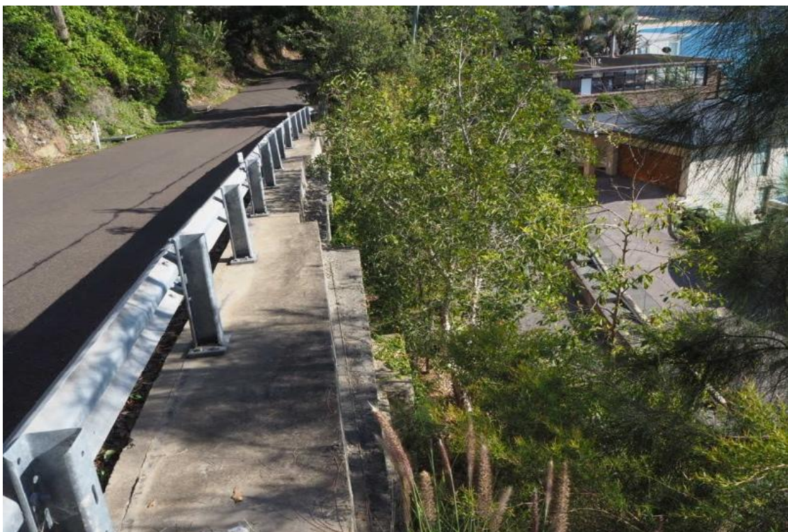
Photo 1: View (looking north) of the top of a newly constructed retaining wall at Whale Beach Site 1
