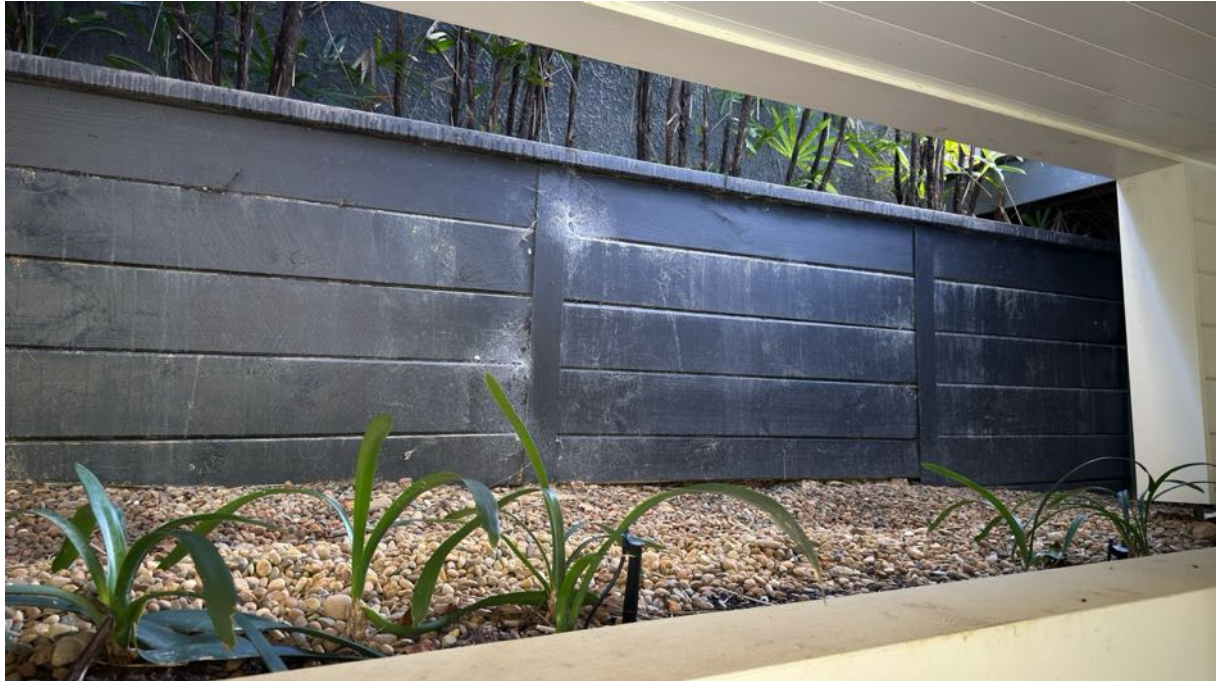
Photo 6 – Closeup view of timber sleeper cantilever wall with steel posts.
