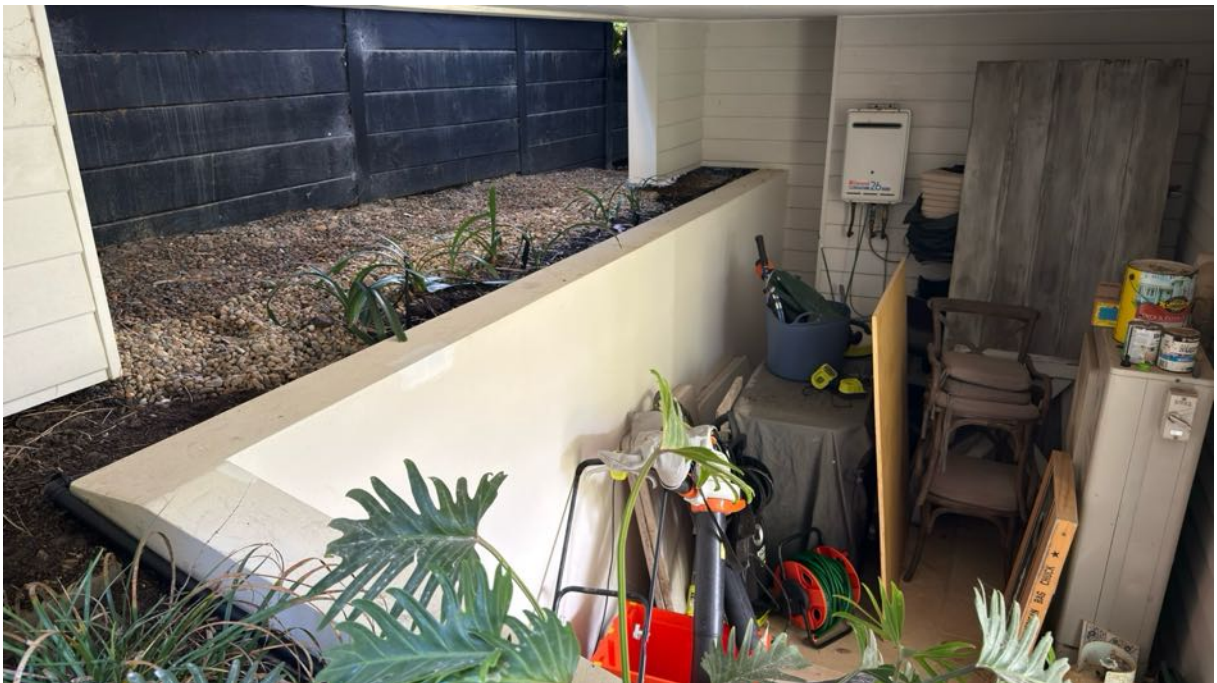
Photo 5 – Rendered concrete wall at lower level of house.
