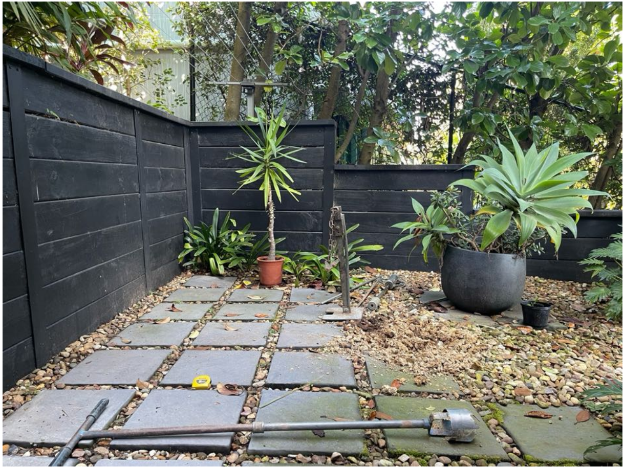
Photo 3 – BH01 Location, note timber sleeper cantilever wall with steel post
