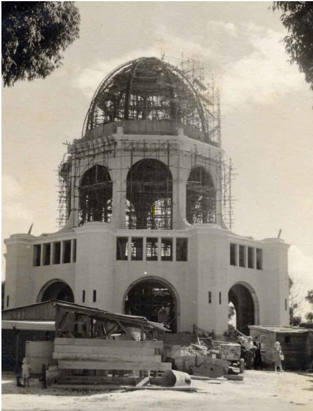
Figure 6 Historical image showing the construction of the Bahá'í Temple which began in 1957. Note: the base form of the dome prior to addition of the lantern to the top via helicopter.
