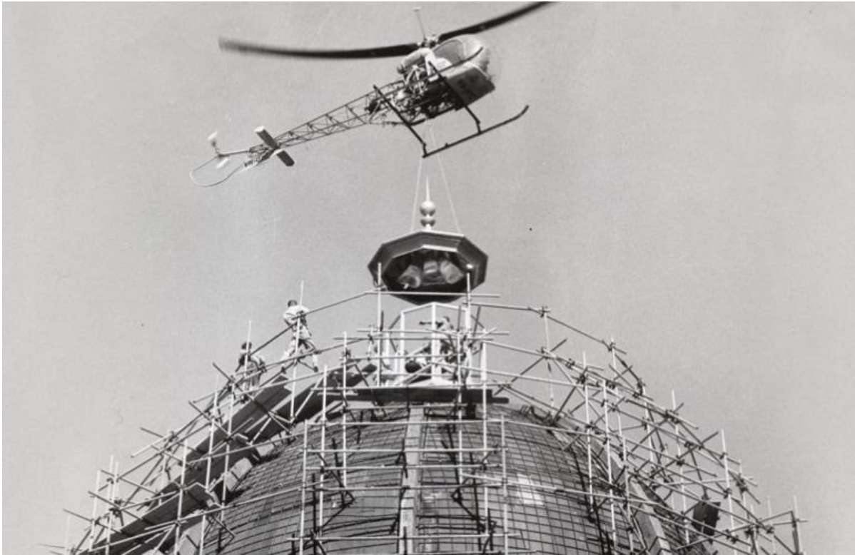
Figure 8 Historical image showing the placement of the lantern atop the Temple's dome via helicopter.
