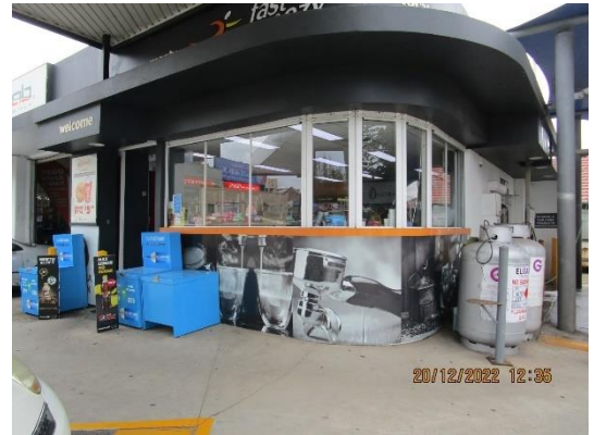
Photograph No. 04 Existing shopfront - to be replaced
