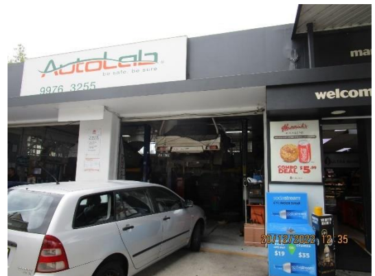
Photograph No. 06 Existing workshop bay - New shopfront for extended sales area
