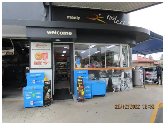
Photograph No. 05 Existing shopfront + door to be replaced
