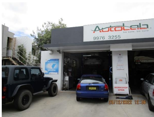
Photograph No. 07 Existing workshop bay - New car wash entry
