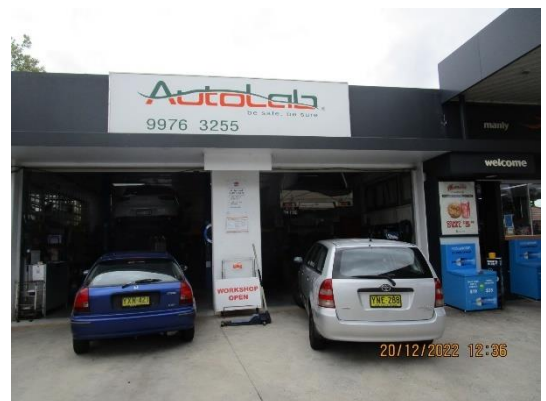
Photograph No. 08 Existing workshop bays - New shopfront on right, new car wash entry on left
