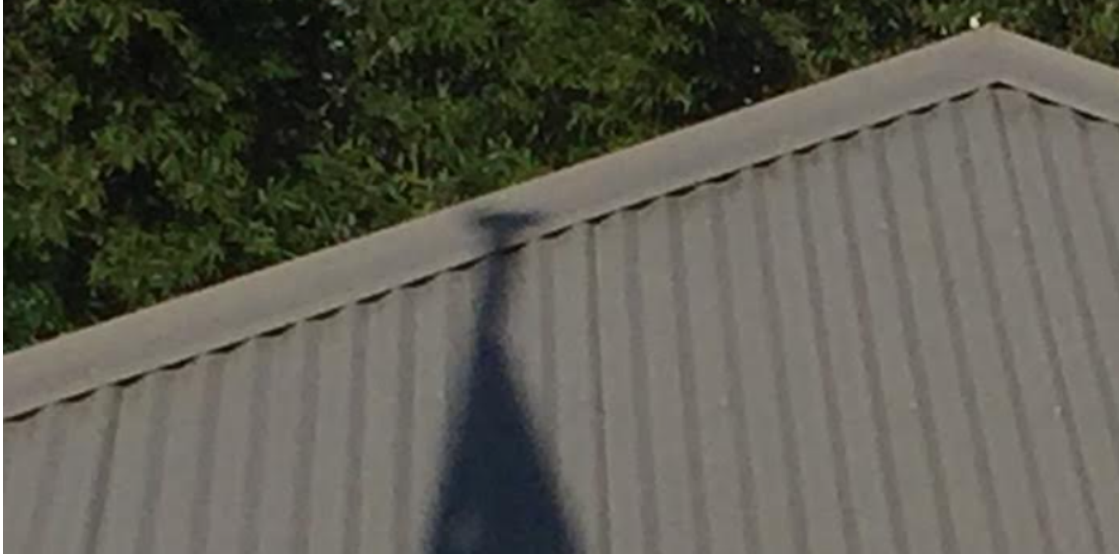
Roof Sheetnig – Colorbond Medium finish
