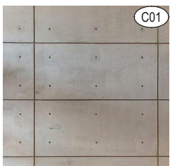
OFF FORM CONCRETE
