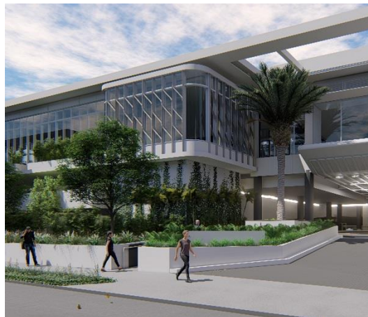
Figure 6a. Revised design for entrance with mullion blades modified into a screen
