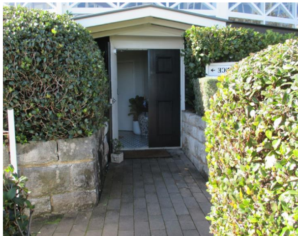
Figure 5- Entry door to the restaurant lobby via the path
