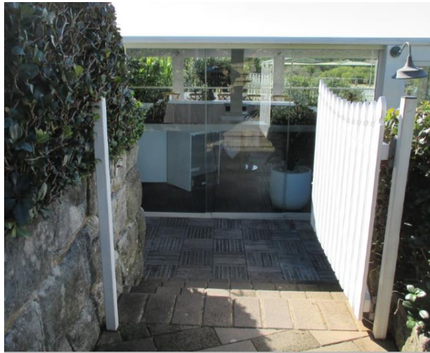
Figure 4- The entry to the pavilion building via steps
