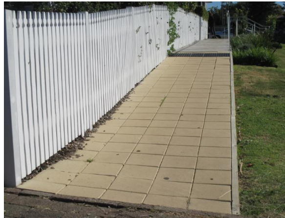
Figure 7- Ramp and walkway access to the coffee shop
