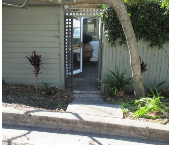
Figure 6- The entry with a steep ramp
