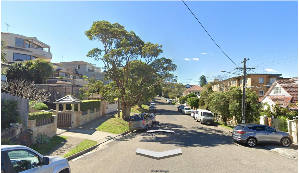
Figure 4: View looking west past subject site on Clifford Avenue
