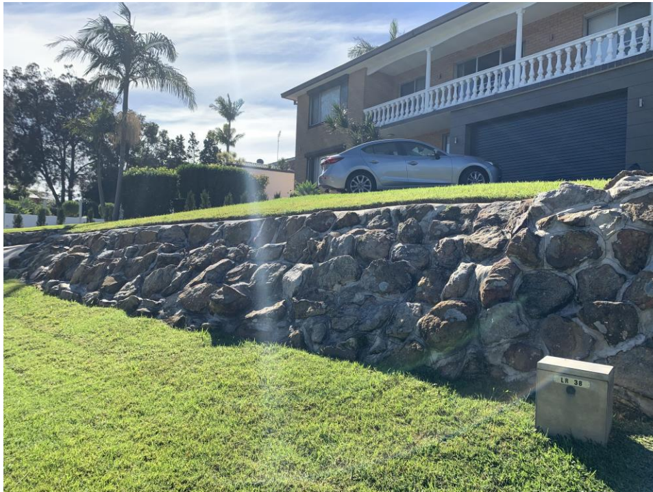
Subject premises and existing bush rock retaining wall to front setback.
