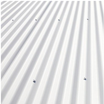
Met1 High quality Colorbond metal sheet roofing, Surfmist or similar
