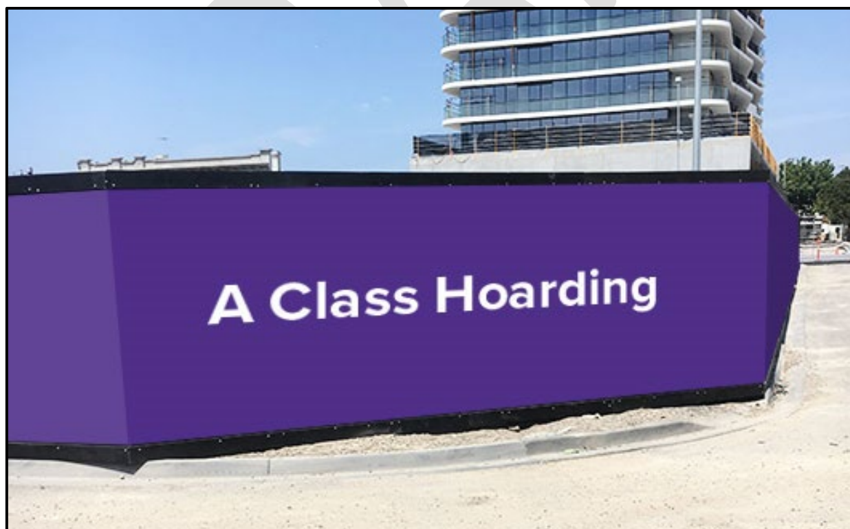
A Class hoarding recommended for Site.
