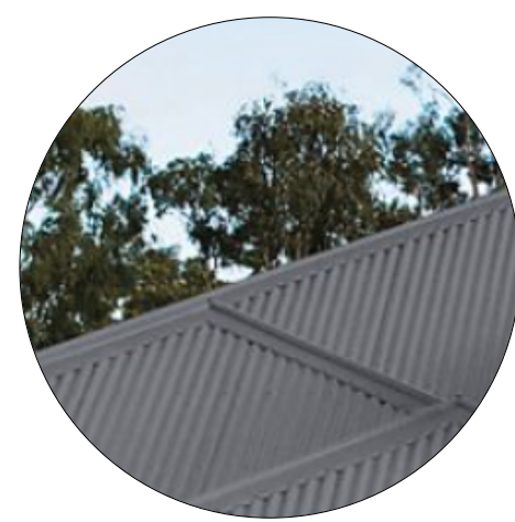
02 CORRUGATED METAL ROOF CLADDING BASALT COLOUR - COLORBOND
