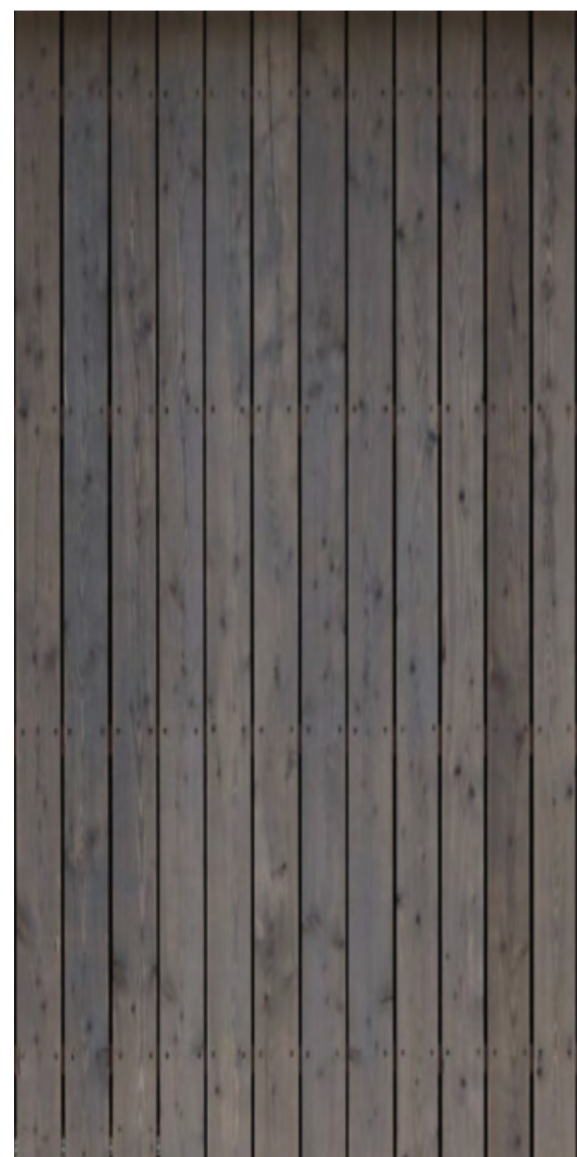
NATURALLY WEATHERED TIMBER CLADDING
