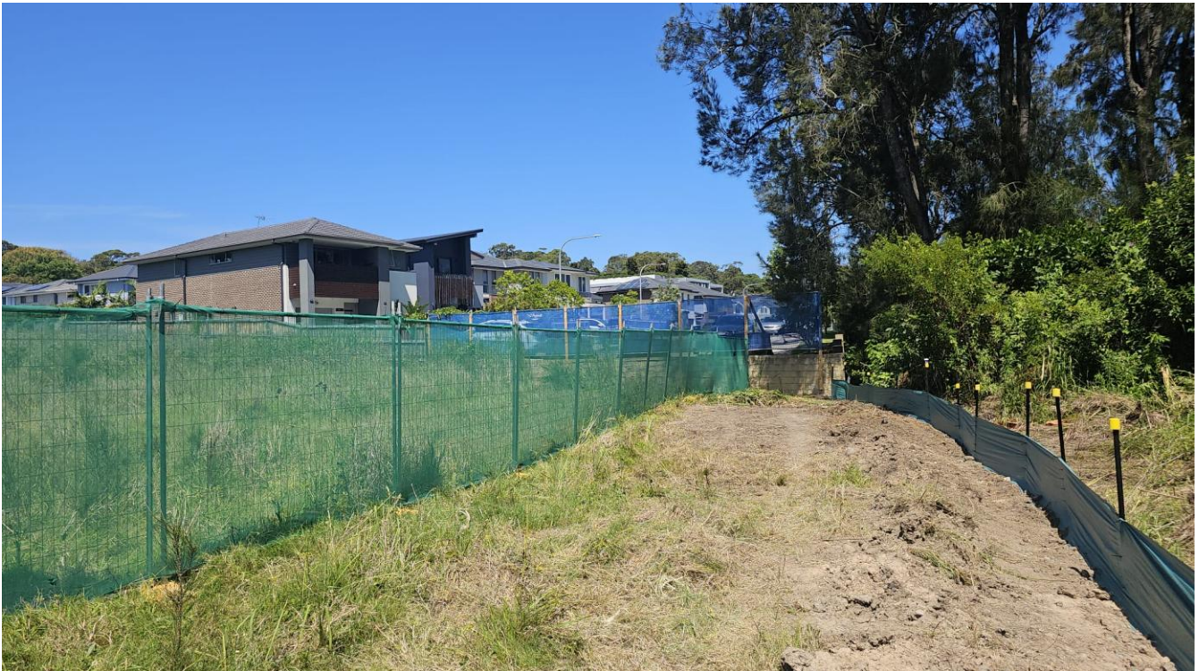
Protection fencing and sediment fencing. Restoration vegetation seen on the right.
