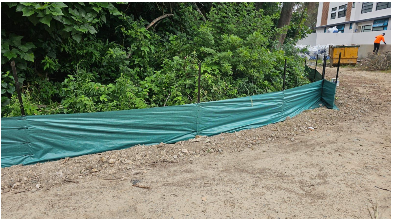
Sediment fencing protecting restoration area.
