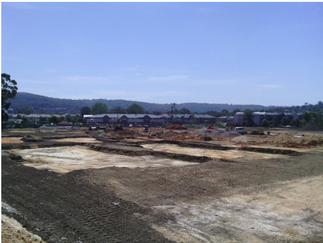
Plate 4. View of construction site to the west
