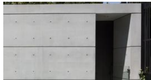
F03 : EXPOSED PRECAST CONCRETE PANEL
