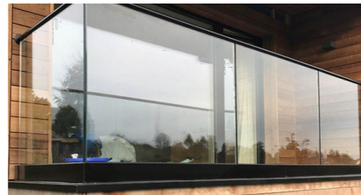
F06 : CLEAR GLAZED POWDERCOATED EQ. DULUX COLORBOND MONUMENT
