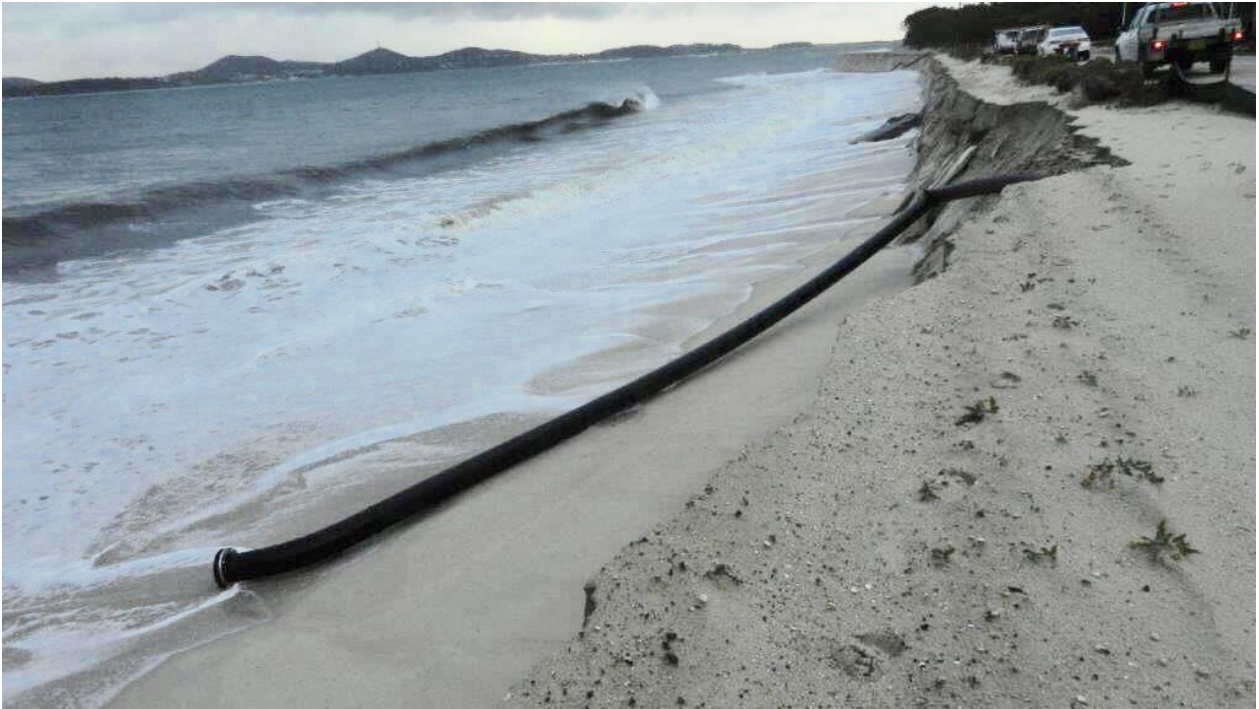
Figure 6-5: Damage to Jimmys Beach sand transfer system by large swell in 2019 (Source: Newcastle Herald, 5 June 2019)
