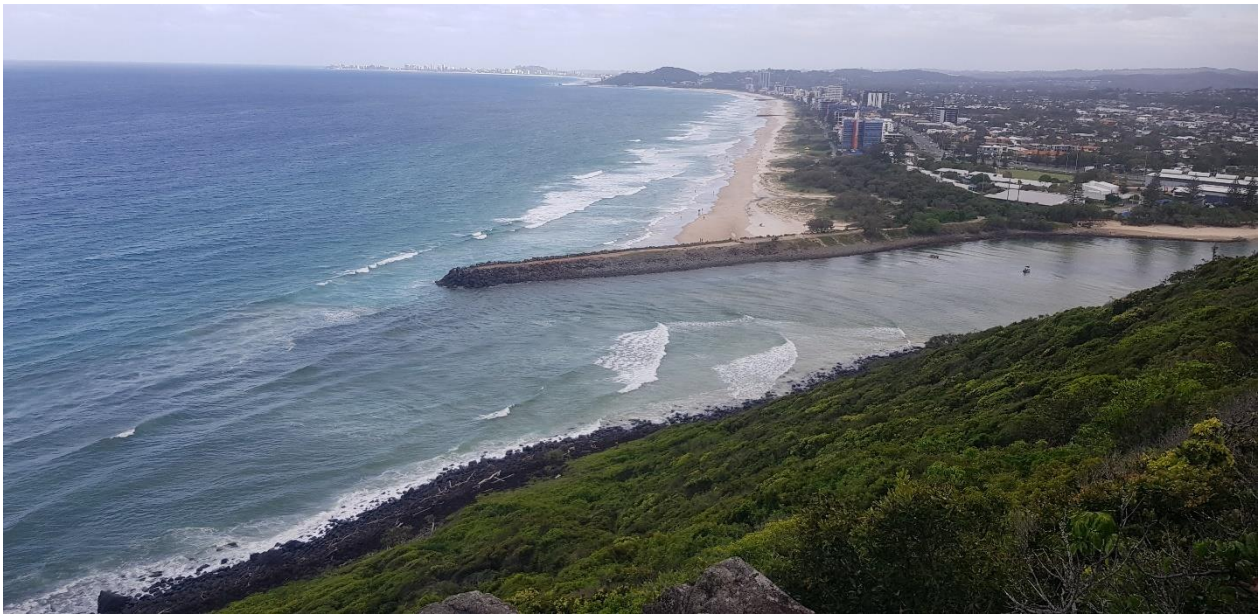
Figure 6-1: Example rock training wall at Tallebudgera Creek entrance
