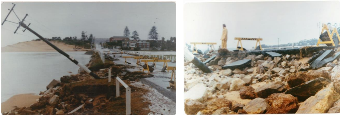
Figure 2-12: Damage to Ocean Street Bridge in 1974
