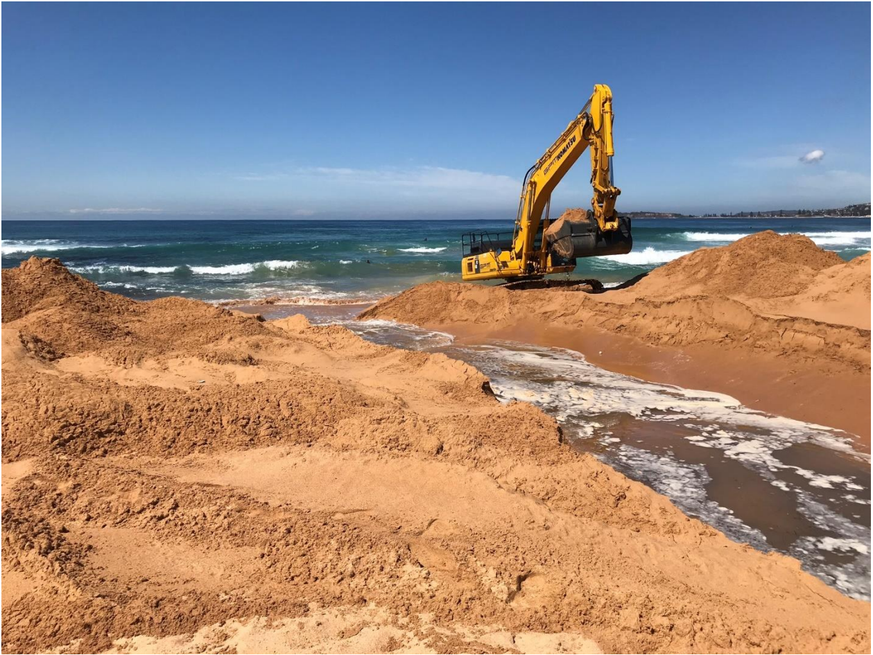
Figure 4-1: Pilot channel excavation, September 2018
