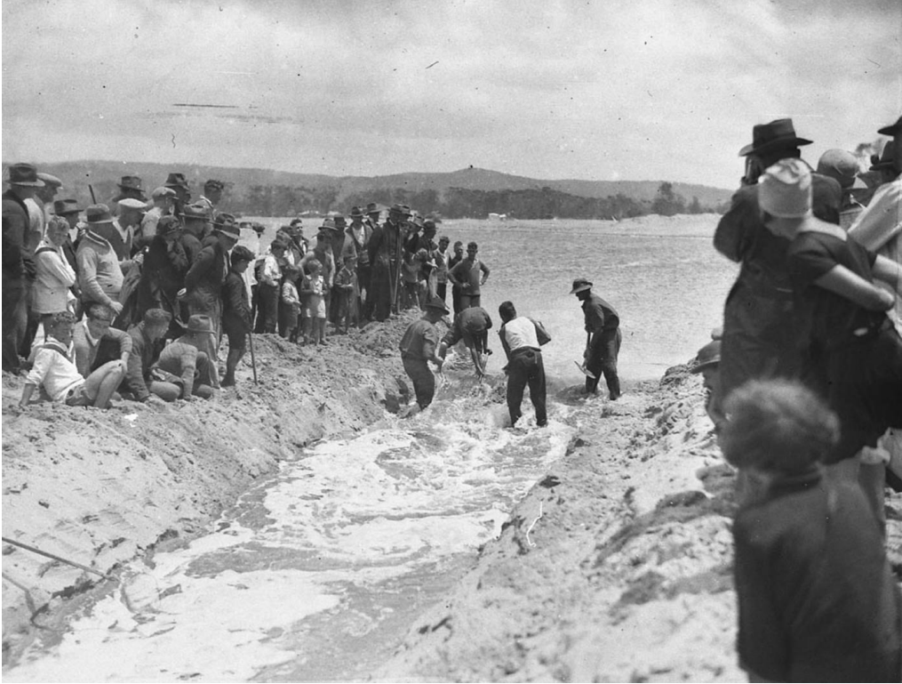
Figure 2-3: Men digging flood mitigation channel, April 1927 (Source: State Library of NSW)
