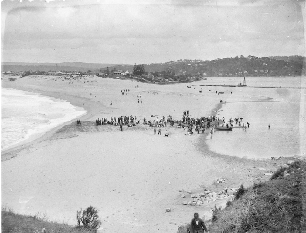
Figure 2-4: View of flood mitigation channel from Narrabeen Headland, April 1927 (Source: State Library of NSW)
