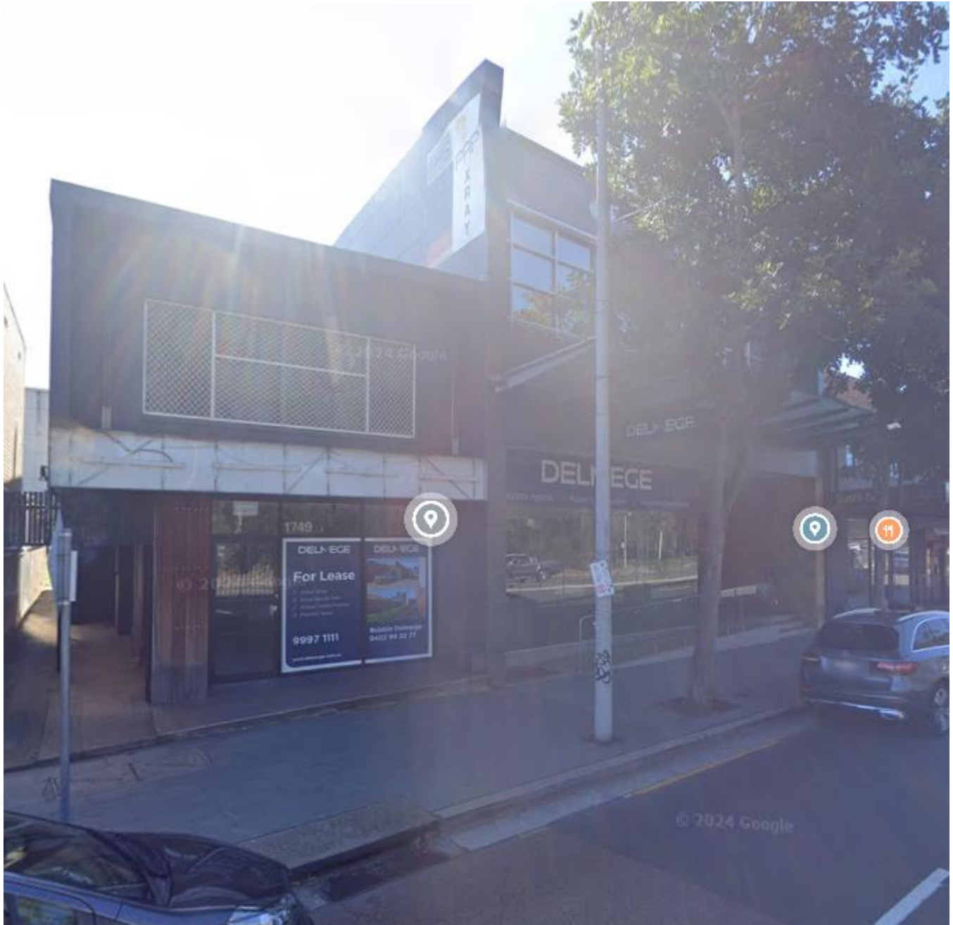
Street view Nos 749 – 1753 Pittwater Rd Mon Vale Note existing building extents on Pittwater Rd frontage to effect flood conveyance (google earth)
