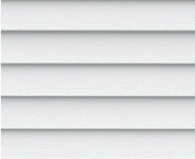
CLD-01 - CLADDING TYPE 01 FIBRE CEMENT CLADDING SIM/EQ TO CEMINTEL WEATHERBOARD 'BALMORAL', PAINT FINISHED SIM/EQ TO DULUX 'NATURAL WHITE'
