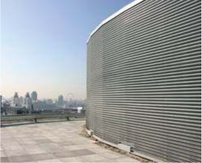
SCR-01 - SCREEN TYPE 01 ACOUSTIC LOUVRE SCREENS, FINISH SIM/EQ TO DULUX 'NATURAL WHITE'
