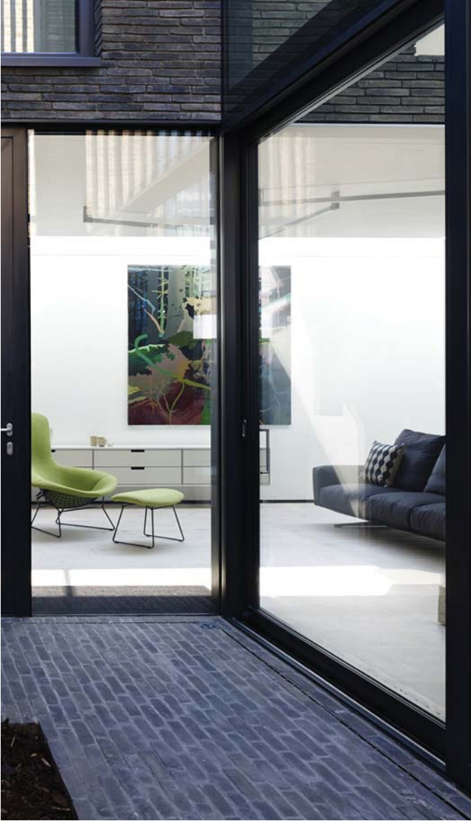
GLZ-01 - GLAZING TYPE 01 CLEAR GLAZING IN ALUMINIUM FRAME, FINISH TO FRAME SIM / EQ TO DULUX POWDERCOAT ZEUS 'BLACK MATT'
