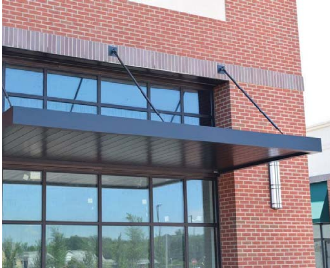
AWN-01 - AWNING TYPE 01 FOLDED SHEET ALUMINIUM CLAD AWNING, POWDERCOATED FINISH SIM/EQ TO DULUX POWDERCOAT 'MONUMENT'
