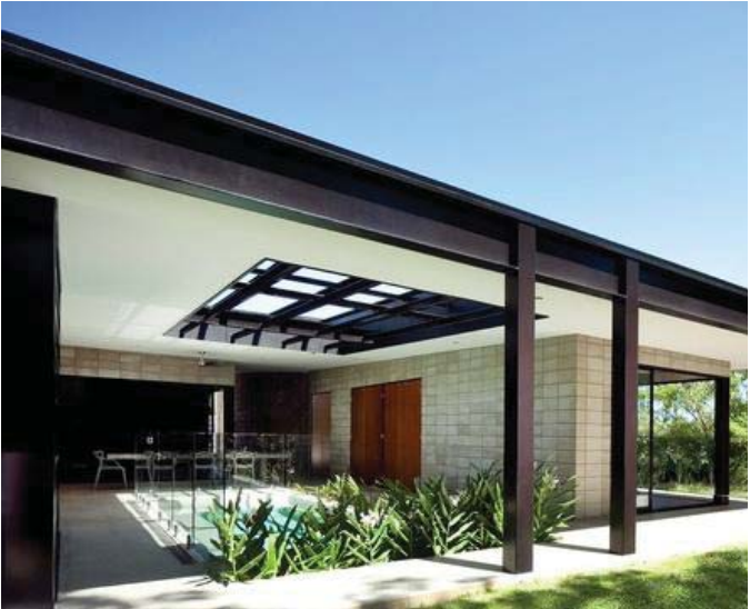
GLZ-02 - GLAZING TYPE 02 SKYLIGHT WITH TINTED GLAZING IN ALUMINIUM FRAME, FINISH TO FRAME SIM / EQ TO DULUX POWDERCOAT ZEUS 'BLACK MATT'
