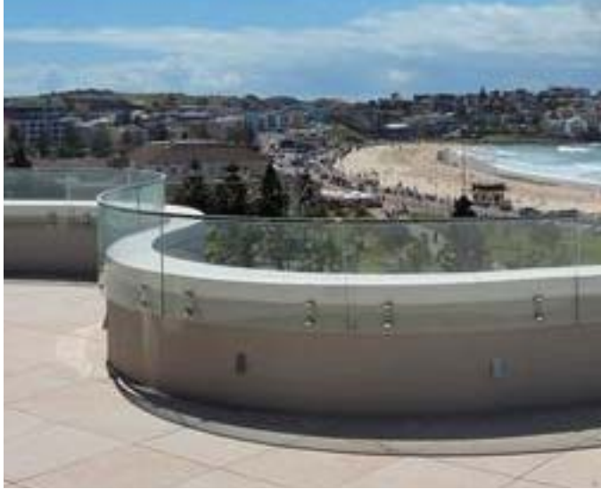
BLD-01 - BALUSTRADE TYPE 01 CLEAR GLAZING BALUSTRADE WITH POWDERCOATED TOP RAIL FIXED TO FACE BRICK PLINTH/RENDERED & PAINTED PLINTH (refer to elevation drawings)
