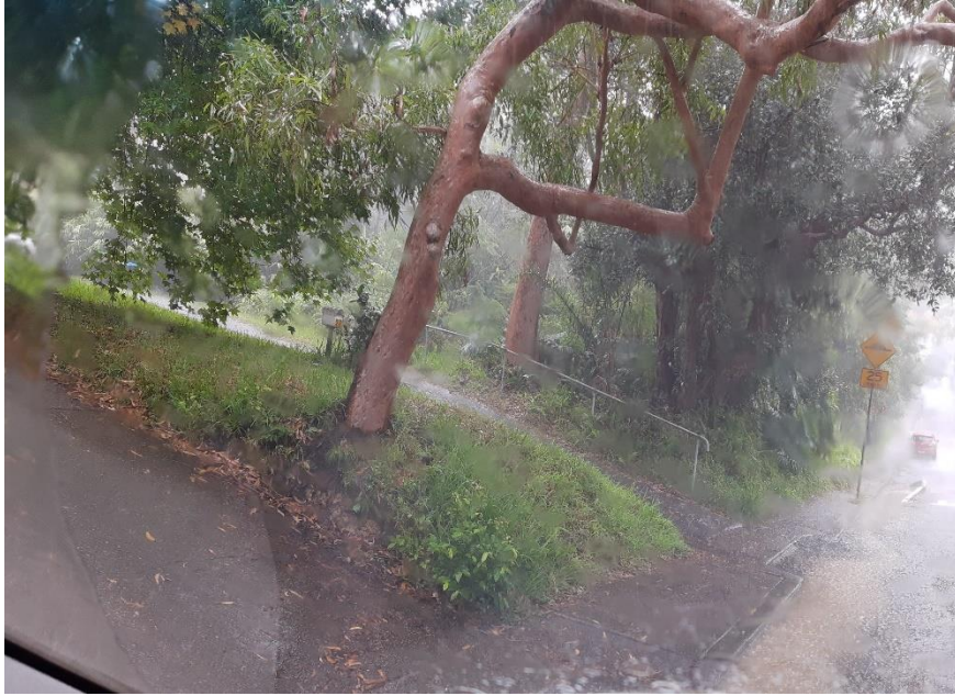
Figure 1 Driveway - showing flooding in light rain & rise from street level
