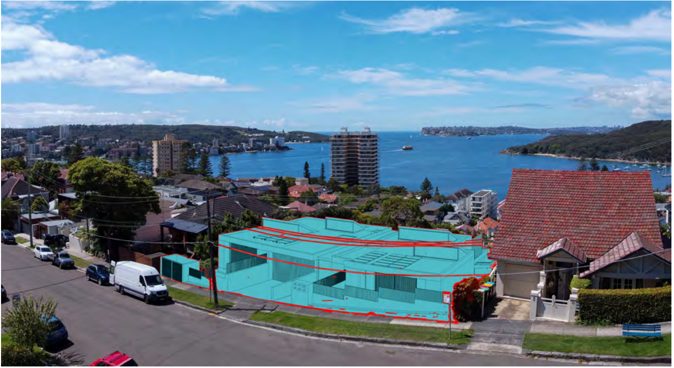
Viewpoint no.20: Visual Impact indicated in red overlay. Visual Quality Assessment: Scale no.13 Visual Impact Assessment: Scale no.2
