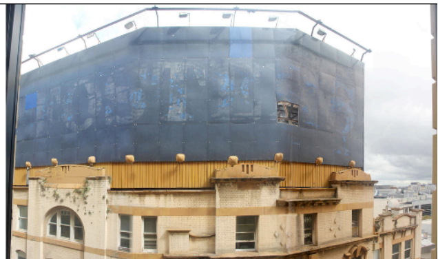
Existing situation – view from adjoining hotel
