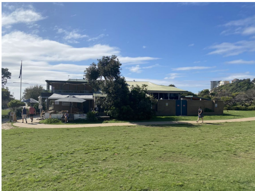
Figure 24: Northwest elevation of the rear addition of the Freshwater SLSC (Source: NBRS, 1 February 2023)
