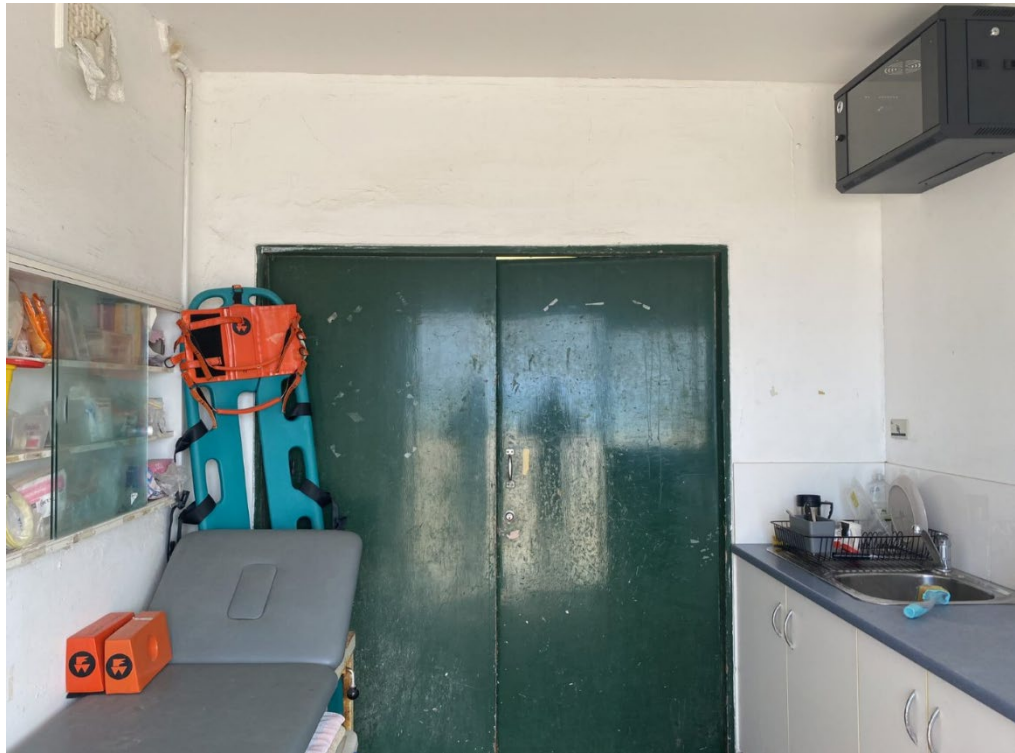
Figure 30: Interior of the first aid room in the eastern corner of the surf club building (Level 1) (Source: NBRS, 1 February 2023)
