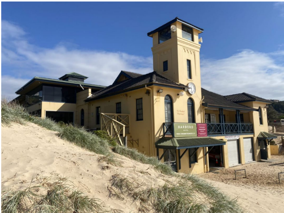
Figure 22: Southwest corner of the Freshwater SLSC (Source: NBRS, 1 February 2023)
