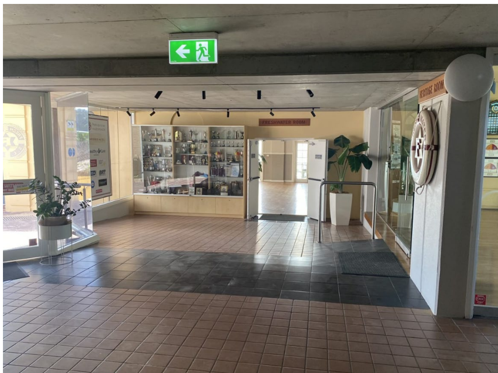
Figure 31: Interior of the junction between the original surf club building and 1980s addition, view looking southeast to the surf club building (Source: NBRS, 1 February 2023)
