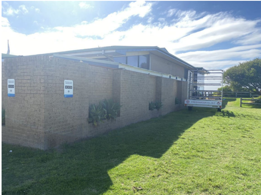
Figure 23: Southwest elevation of the Freshwater SLSC rear addition (Source: NBRS, 1 February 2023)
