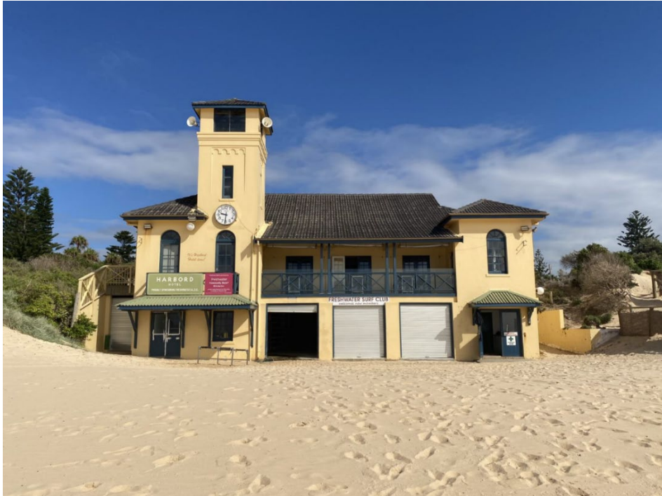
Figure 21: Principal facade of the Freshwater SLSC, view looking northwest from Freshwater Beach (Source: NBRS, 1 February 2023)
