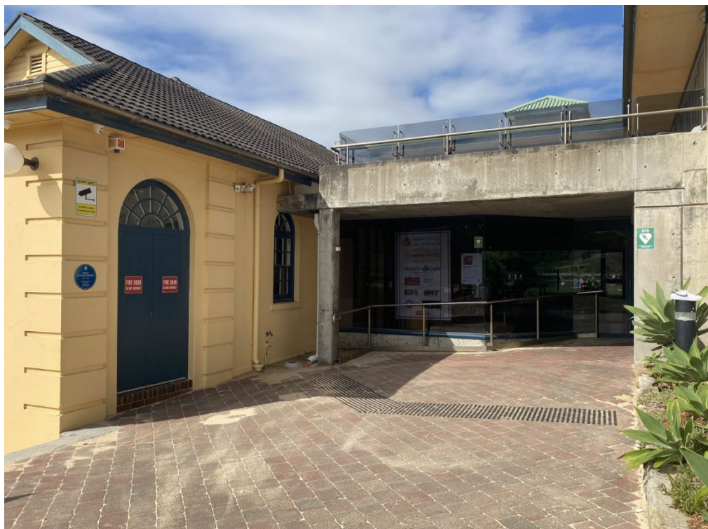
Figure 26: Northeast elevation of the subject site at the central junction between the later 1980s addition to the site (right) and the original 1930s clubhouse (left) (Source: NBRS, 1 February 2023)
