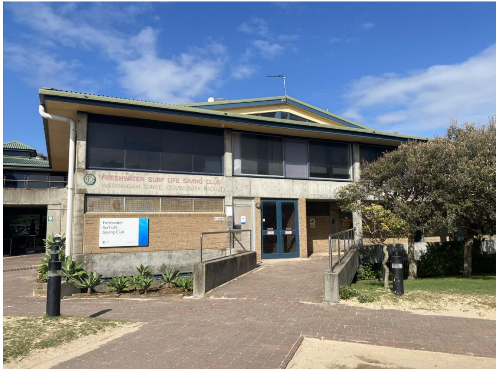
Figure 25: Northeast elevation of the rear addition of the Freshwater SLSC (Source: NBRS, 1 February 2023)
