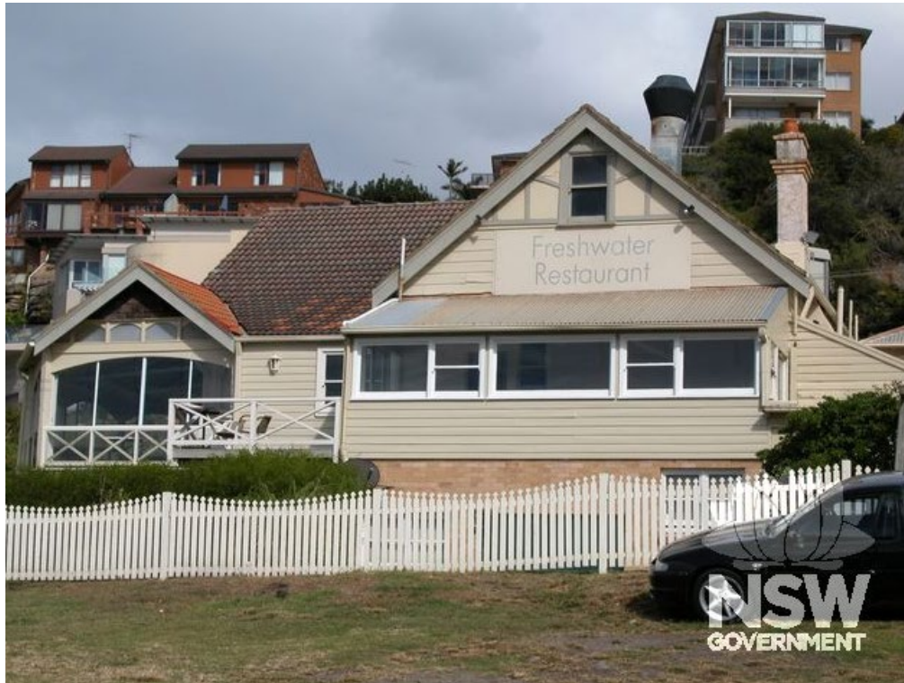
Figure 40: Image of Freshwater Restaurant, July 2020, from the State Heritage Inventory Database (Source: Mayne Wilson & Associates, accessed via https://www.hms.heritage.nsw.gov.au/App/Item/ViewItem?itemId=2610064 )
