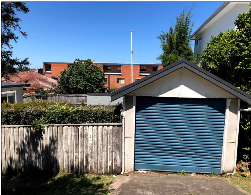
Figure 7: View of Somerville lane from Highview Avenue
