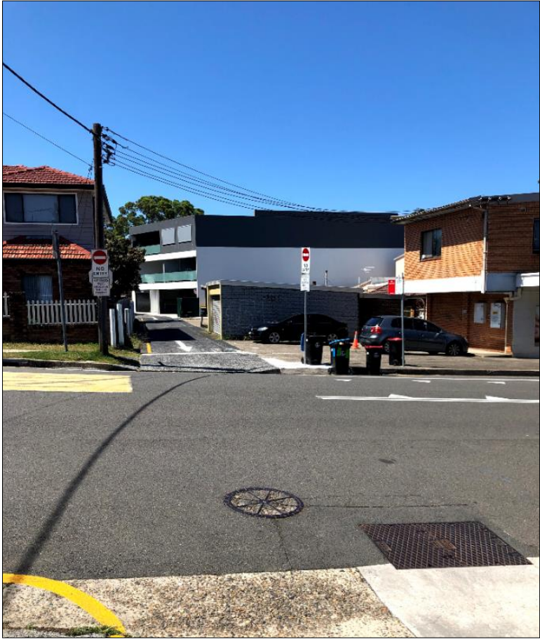
Figure 8: 333 Condamine Street Viewed from Sunshine Street
