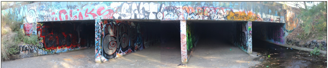
Figure 1: Culvert as viewed from the downstream apron.
