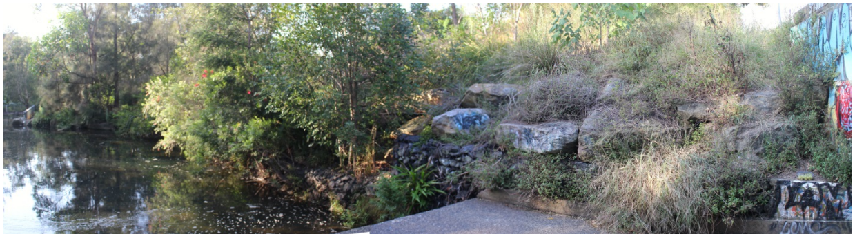
Figure 3: Southern slope to apron
