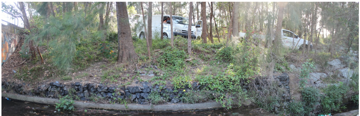
Figure 2: Northern slope to apron
