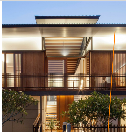
PAINTED TIMBER LINING BOARD EAVES
