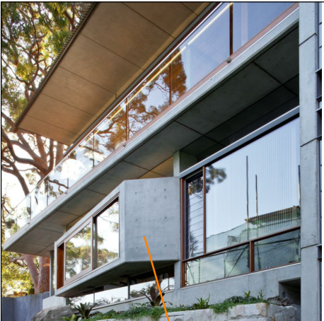
OFF FORM CONCRETE STRUCTURE
