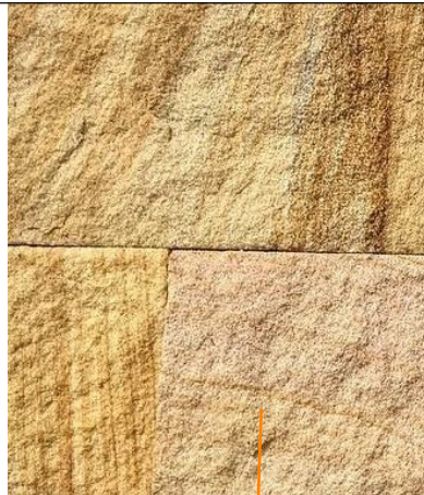
SANDSTONE BLOCK WALLS
