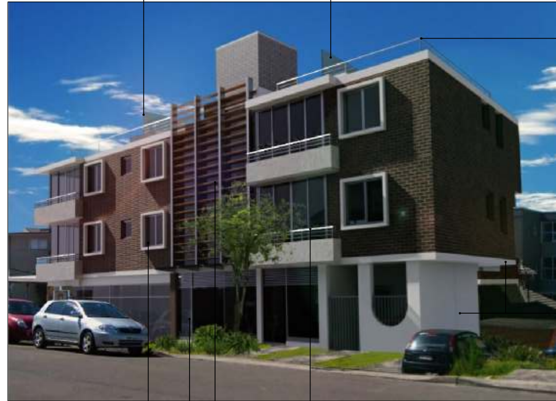
Marine grade stainless tubing & steel wire to perimeter of roof terraces
