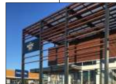
Decowood aluminium louvre beams on vertical frame to stairwell glazing
