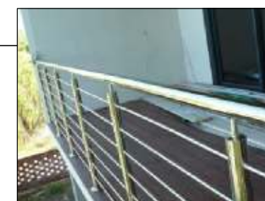
Marine grade stainless steel tubing above cement rendered /paint finished masonry & commercial terrace
