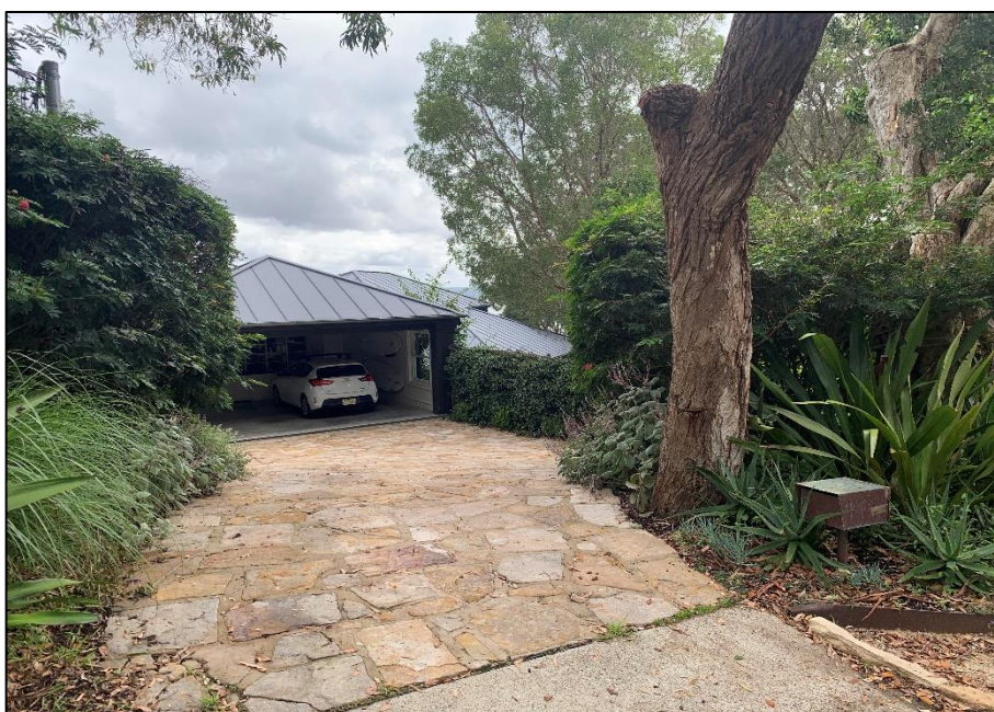
Photograph 2: The driveway and garage, as viewed from the street
