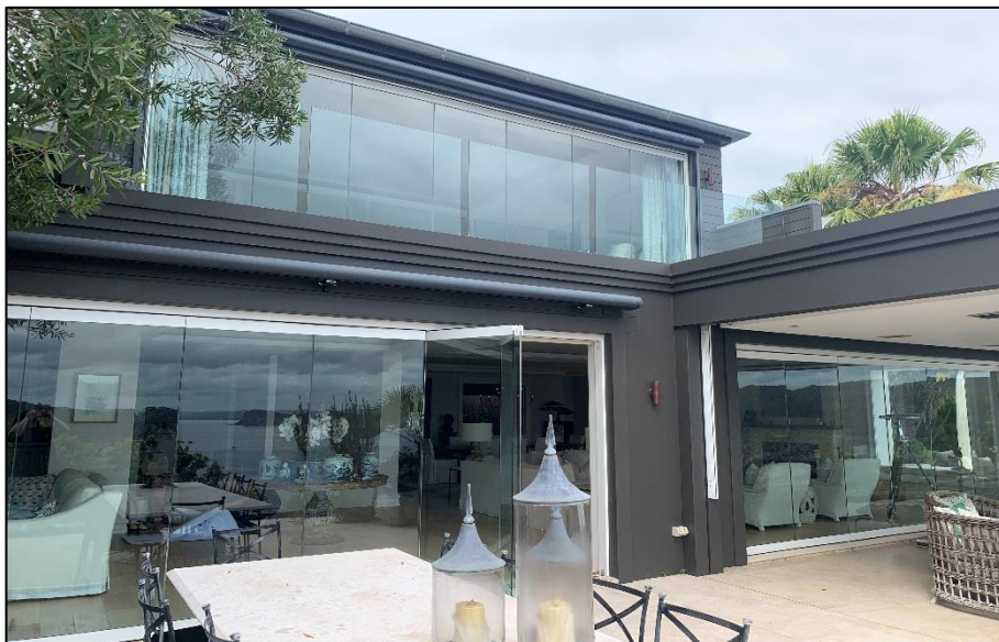
Photograph 4: The rear of the dwelling, as viewed from the outdoor dining terrace
