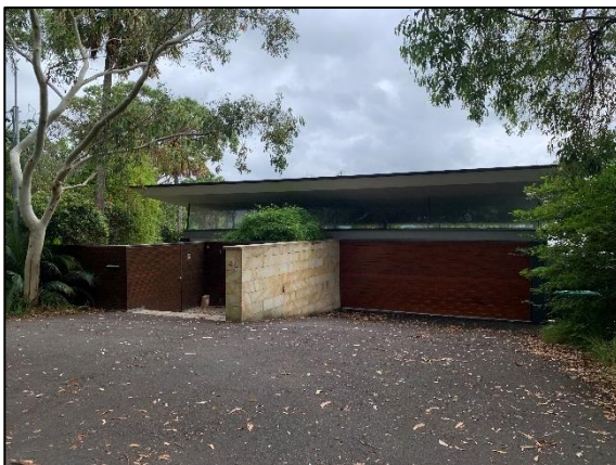
Photograph 10: No. 46 Sunrise Road, as viewed from Sunrise Road
