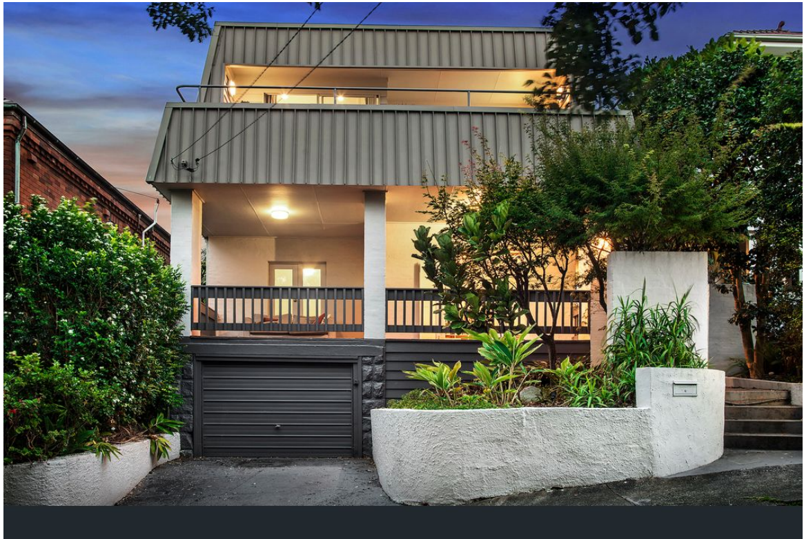
STREET BOUNDARY VIEW OF EXISTING DEVELOPMENT AT UPPER CLIFFORD AVENUE, FAIRLIGHT (shows extremely low head height of existing garage and 83° 'Mansard' style first floor cladding)
