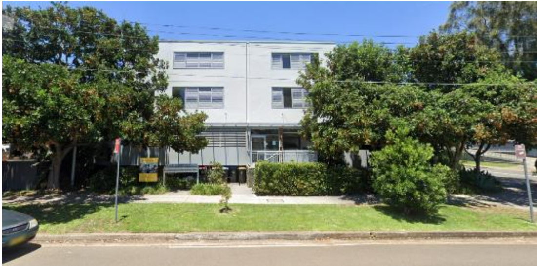
Figure 5: 3 storey shop top housing development at 9-11 Gondola Road
