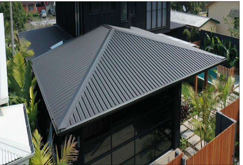
3. COLORBOND MONUMENT METAL ROOF
