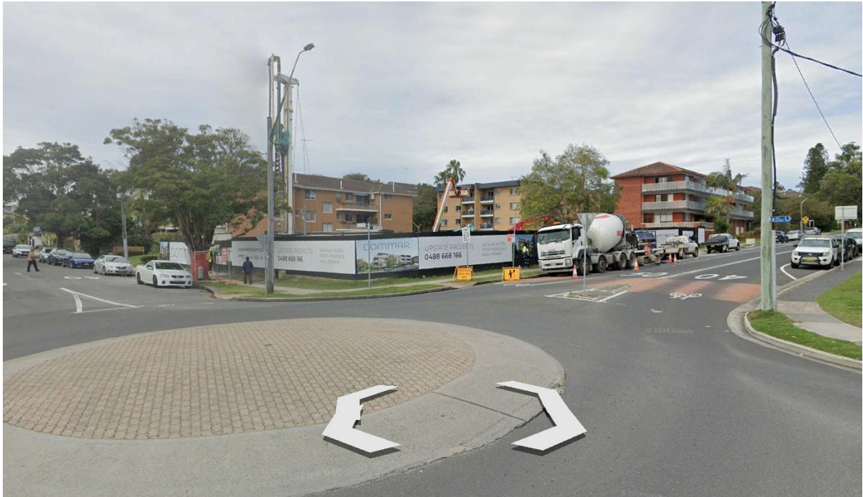
Figure 7: View looking south-east from site towards existing 4 storey residential flat buildings including the 4r storey residential flat building currently under construction on the opposite corner
